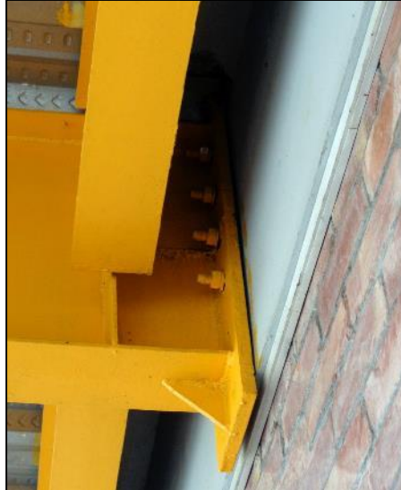
Improper connection
