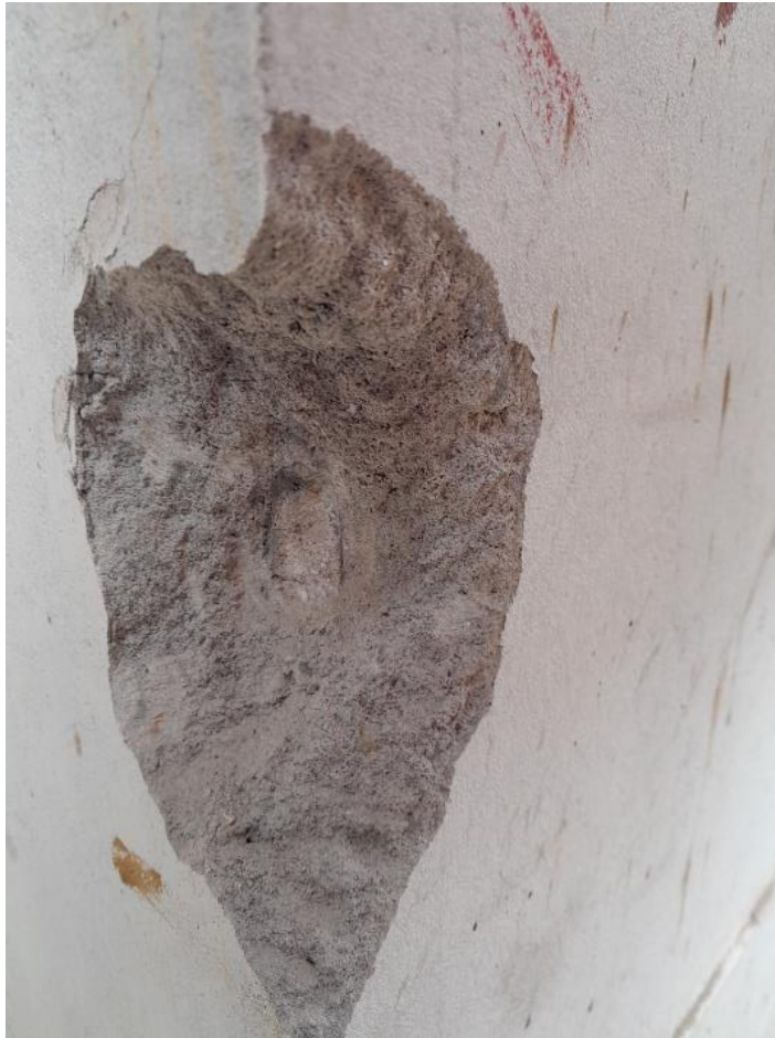
Stone chips aggregate concrete in the column of ETP Building
