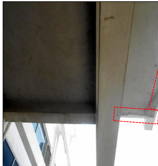
Beam missing on site
