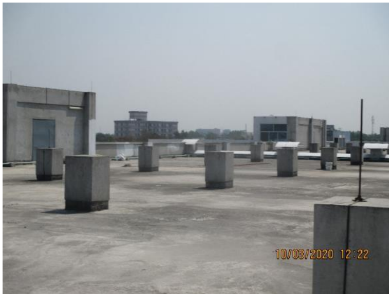
Current roof of factory building
