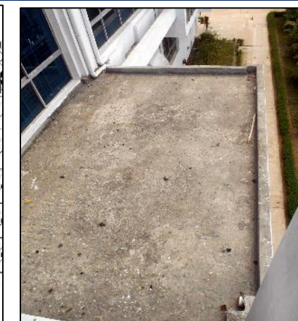
Extra slab on 1 st floor
