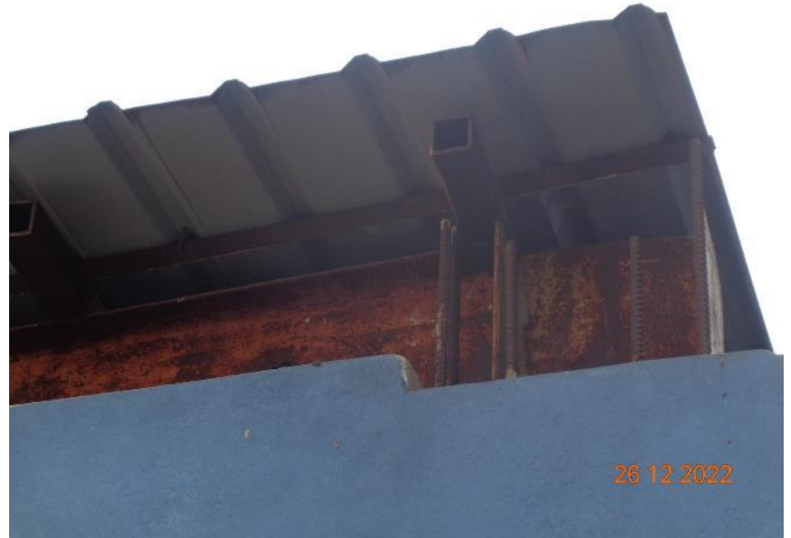
Corrosion in the steel beams
