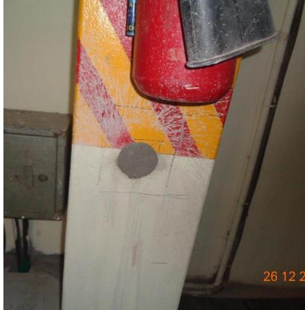
Concrete core taken from column
