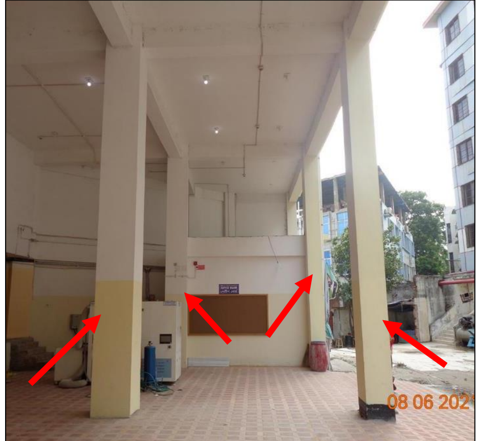
Columns having no barrier/protection at ground floor
