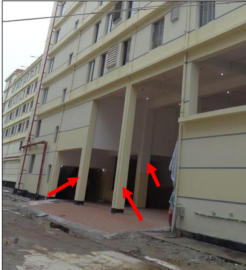
Columns having no barrier/protection at ground floor
