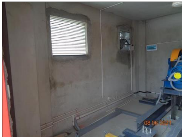
Lift machine room wall is constructed by brick
