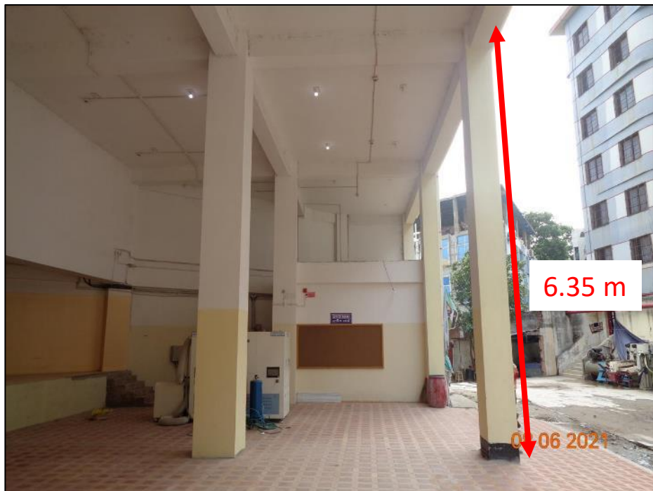
Column at loading-unloading area.
