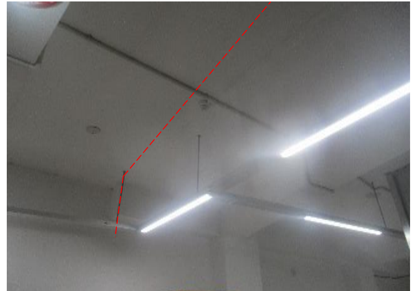
Expansion Joint (1st & 2nd floor only)
