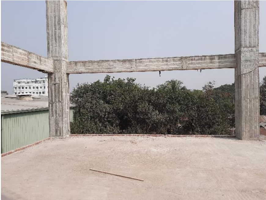
No edge protection provided on roof
