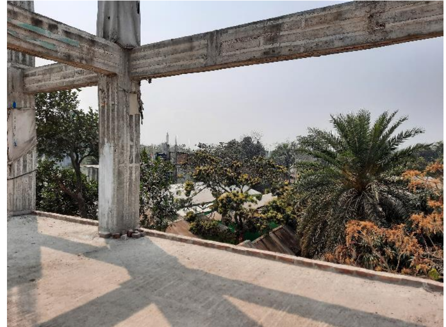
No edge protection provided on roof
