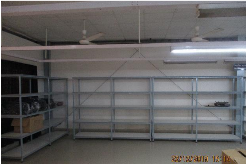
Loose cable bracing
