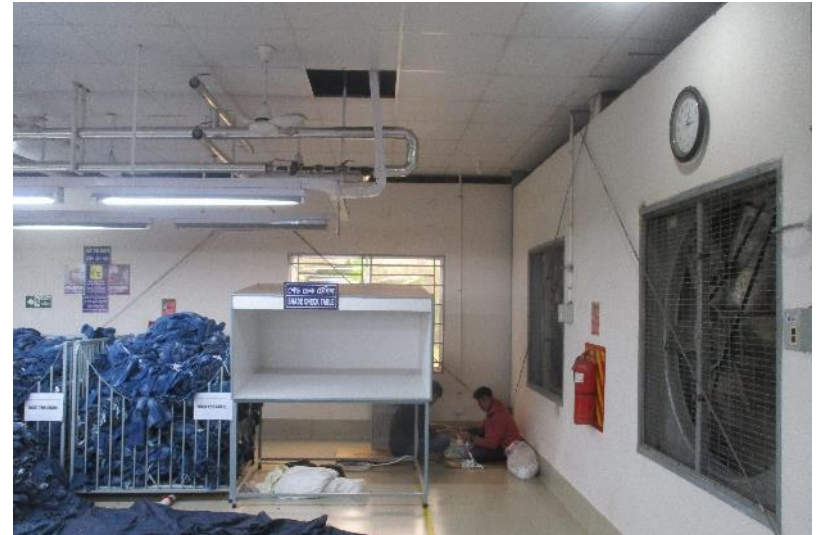
Loose cable bracing
