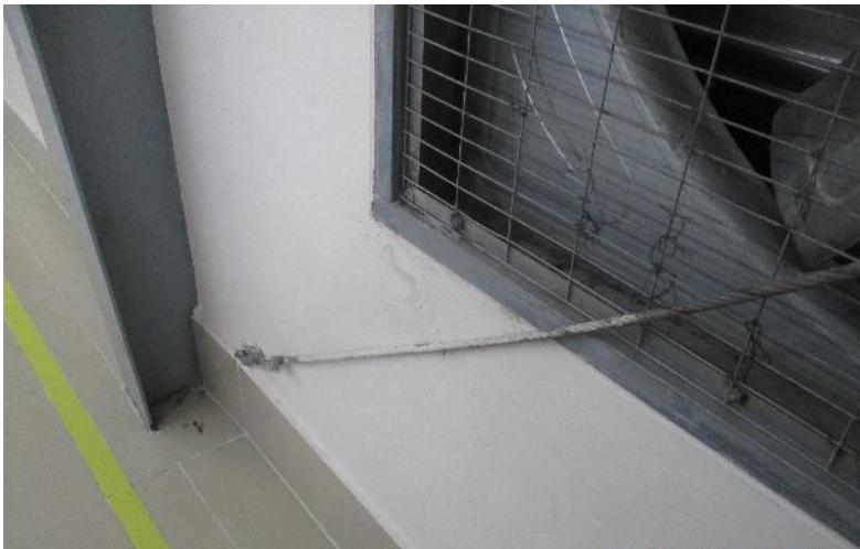
Wall bracing connected to façade wall (non-engineered)
