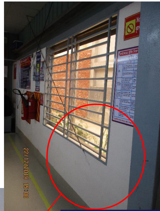
Improper connection of wall bracing
