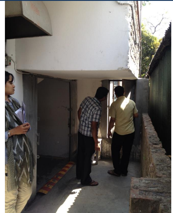
West stair cantilever.
