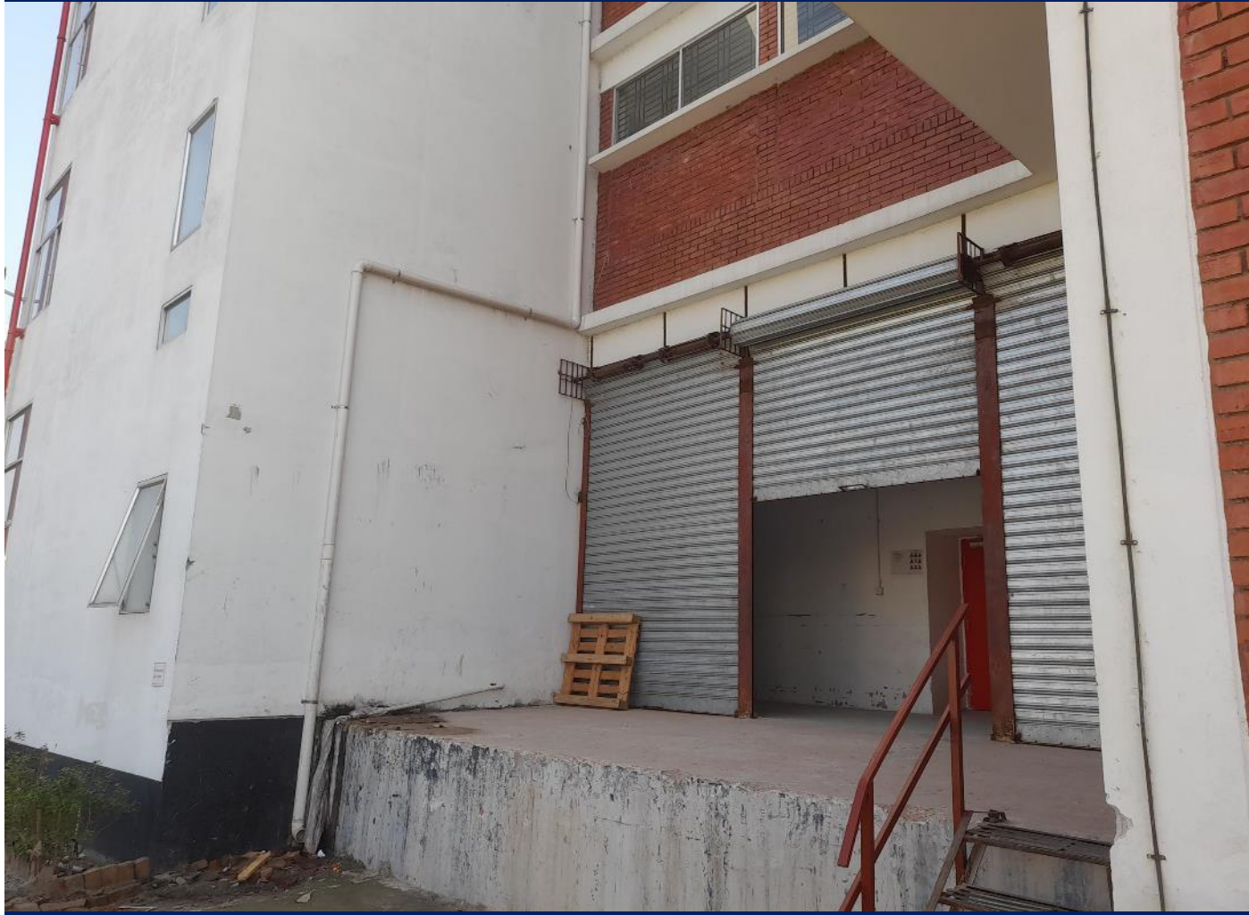
Column at loading/unloading bay
