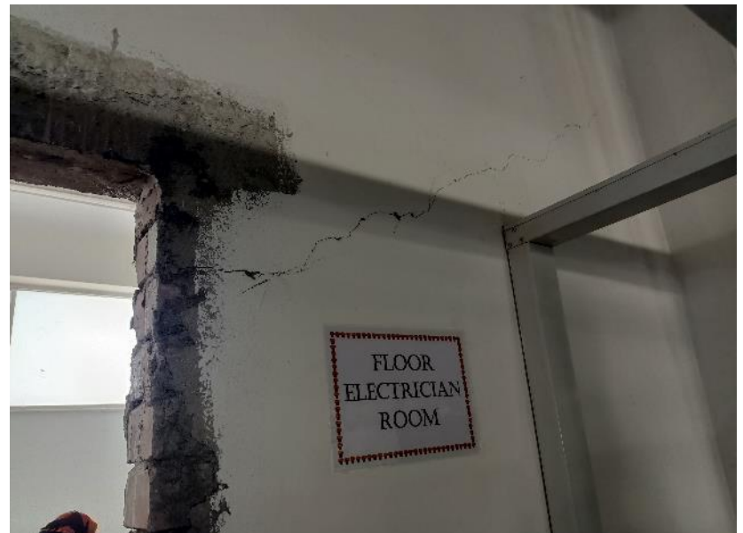
Cracks on brick wall in several location on 2nd floor
