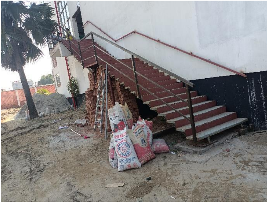
External steel stair at East
