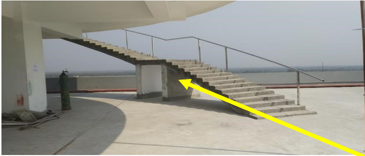
Stair (Roof to Helipad) supported by two brick wall, but one brick wall is shown in drawing
