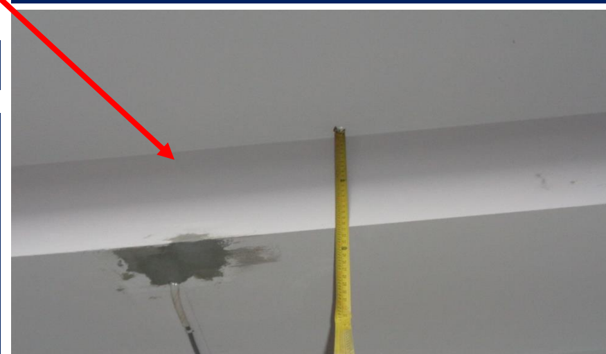
Depth of the beam measured 525mm d/s
