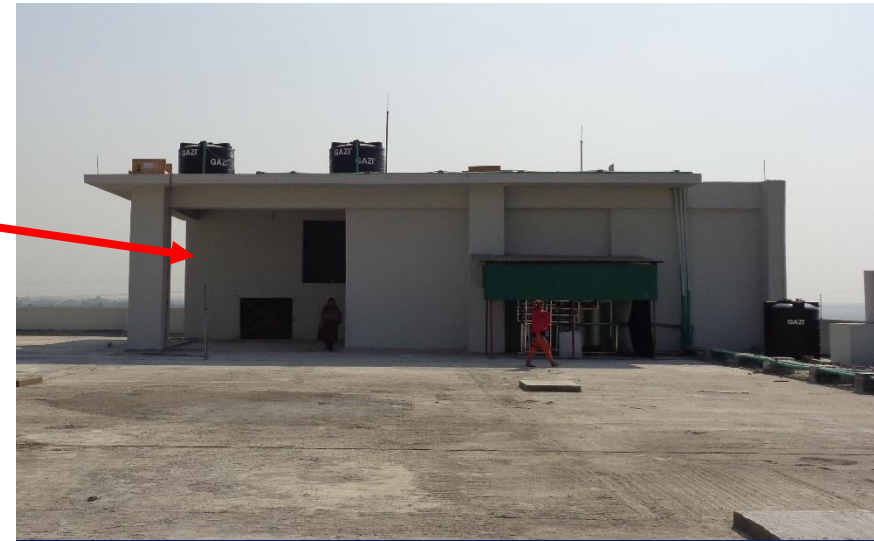
Stair room at south west side
