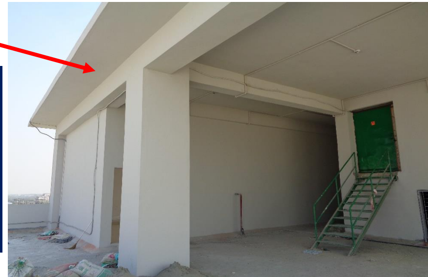
Stair and lift area at south east corner
