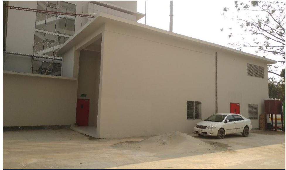
No design report was available for Boiler Building
