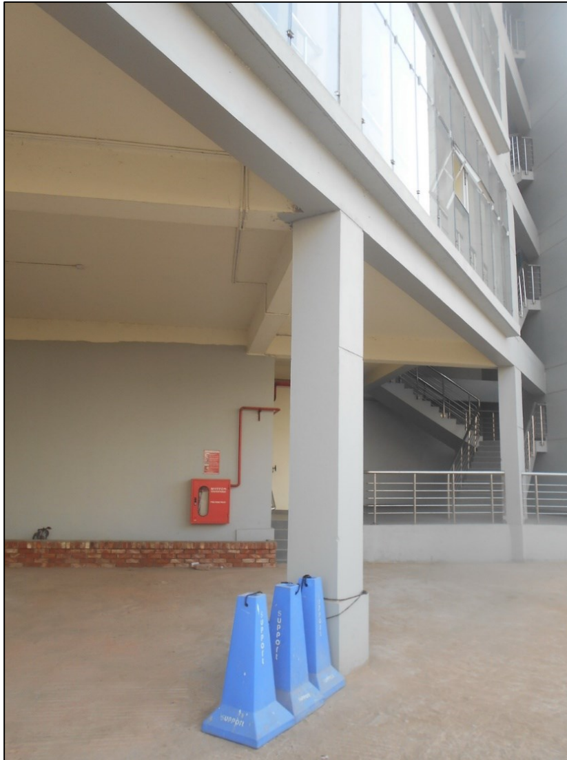
Column of admin building on ground floor
