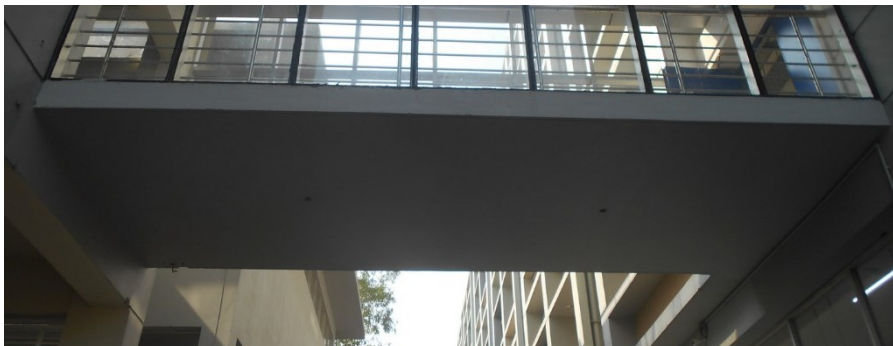
Slab of connecting bridge
