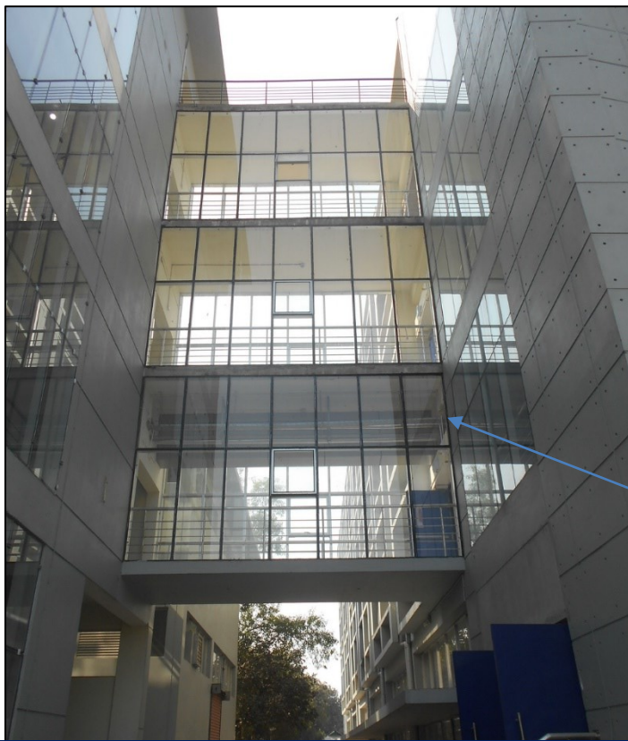
Connecting bridge between production building and store building
