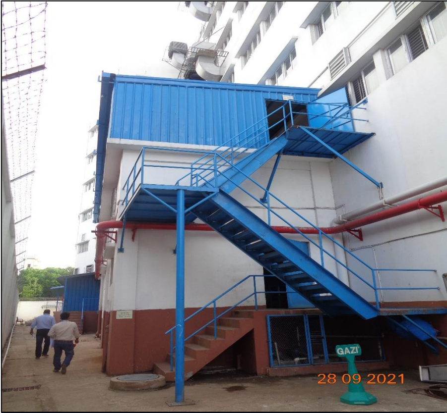
External Steel Stair
