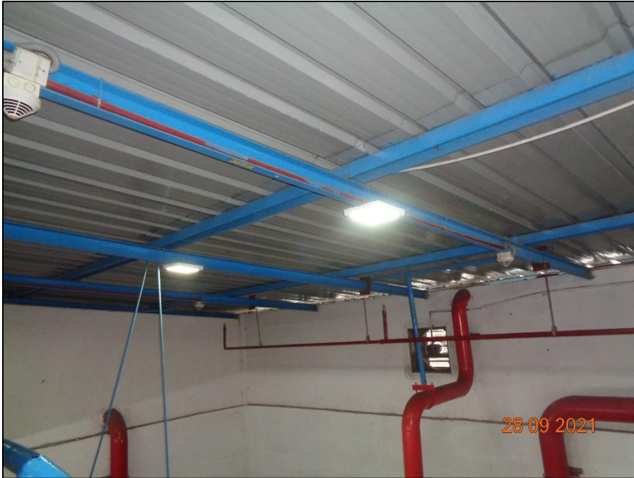
Light weight roof supported on peripheral wall
