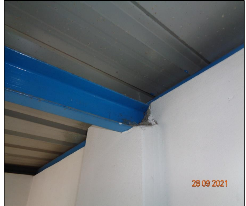
Non-engineered connection
