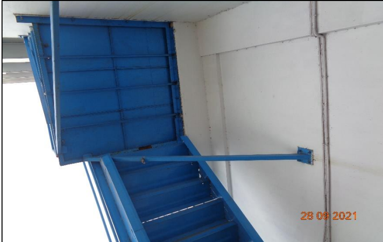
Support System of Steel Stair
