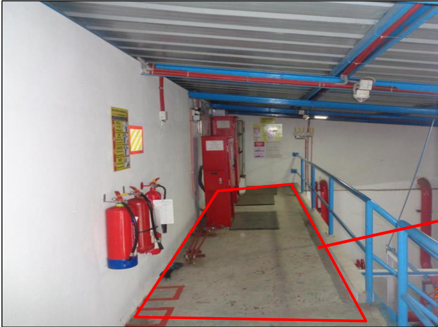
Cantilever slab in pump room
