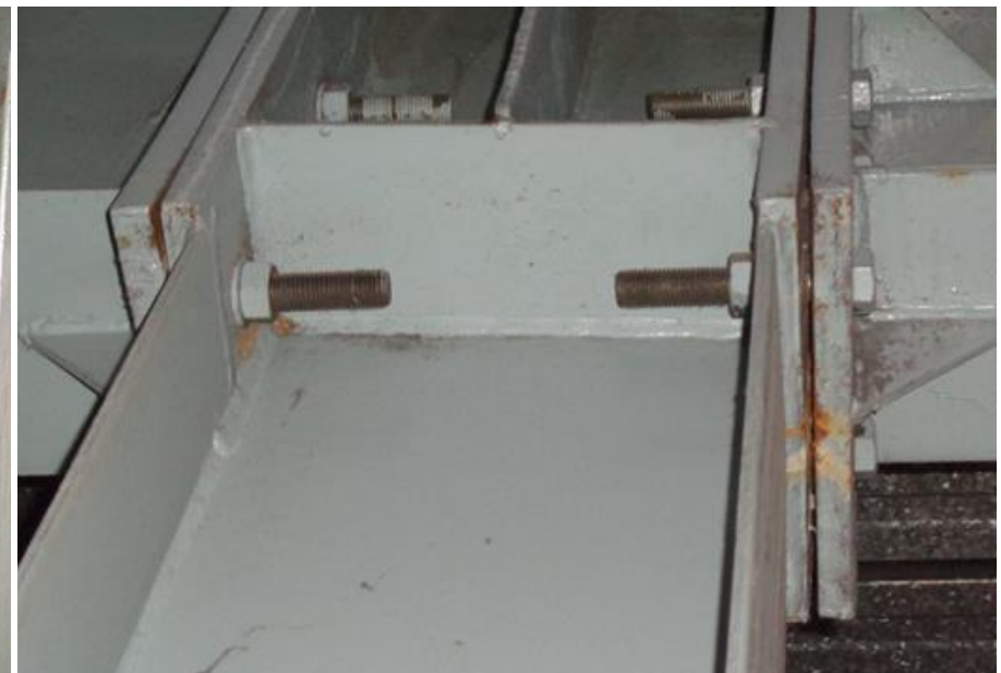
Gap observed in Beam- Column connection
