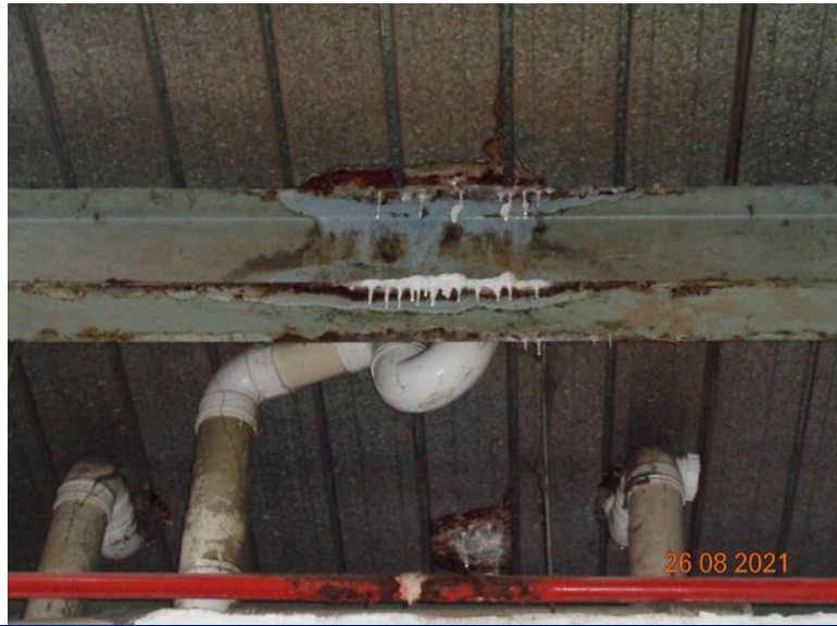
Corrosion in steel beam, column & beam-column connections
