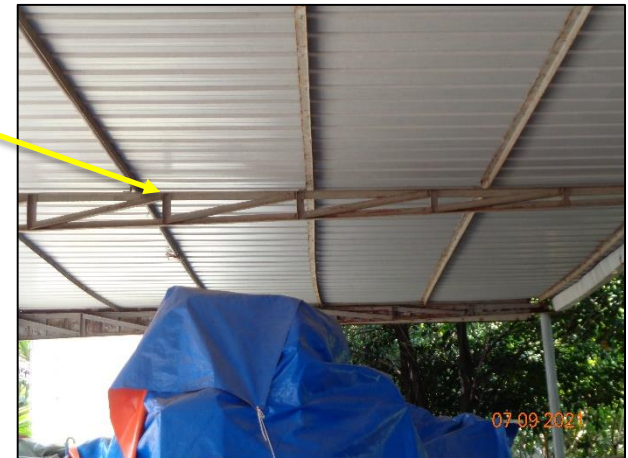
Truss orientation on-site
