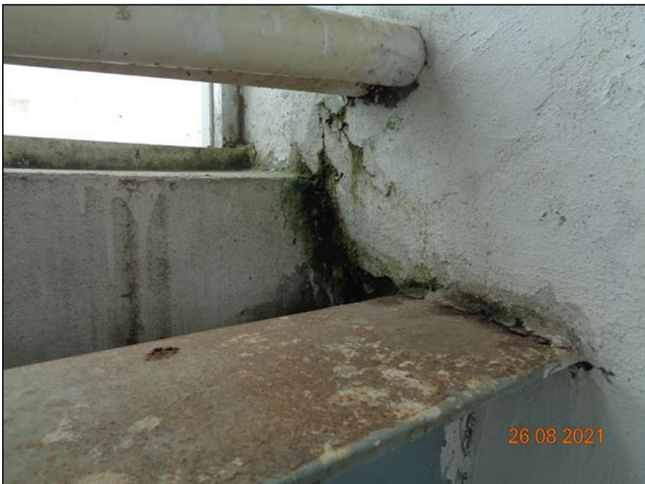
Dampness found in brick wall.
