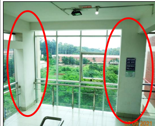
Orientation of marked column found mismatched
