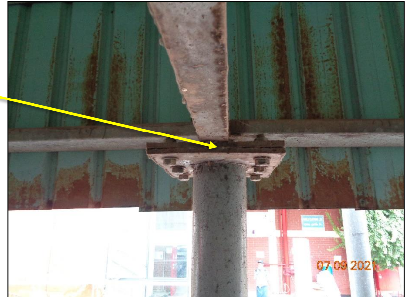
Steel pipe to truss connection
