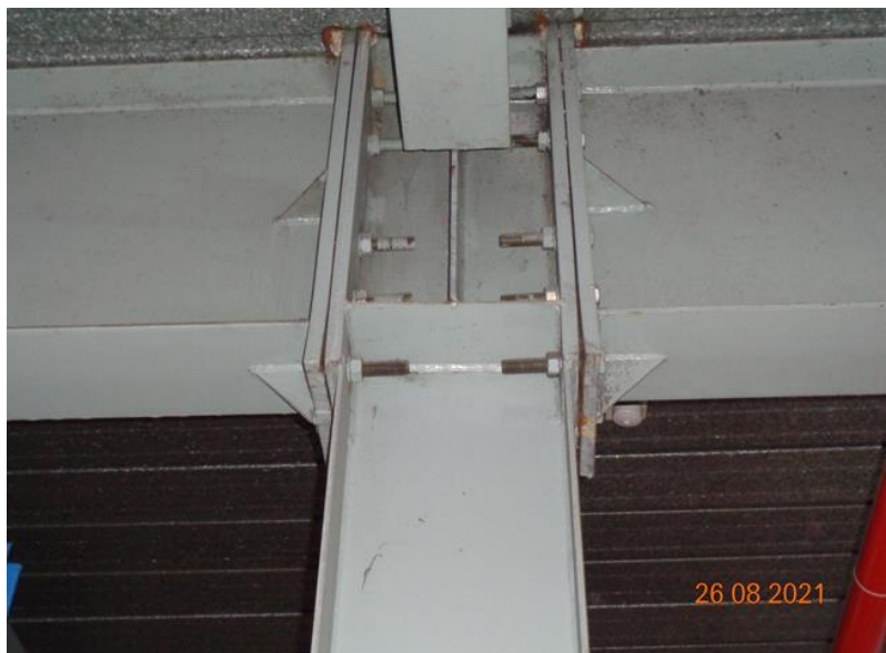
Beam-Column Connection
