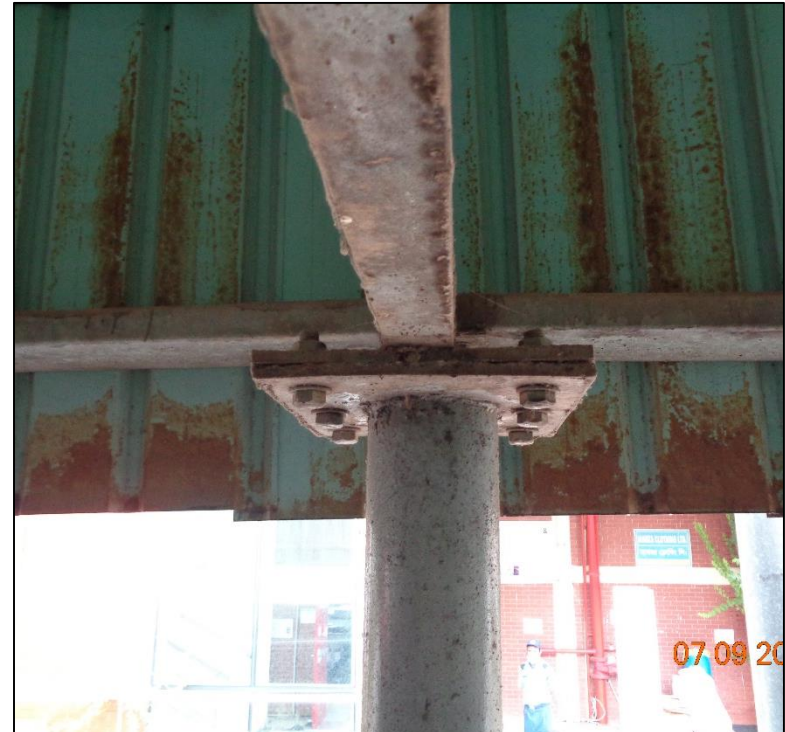
Corrosion in steel column
