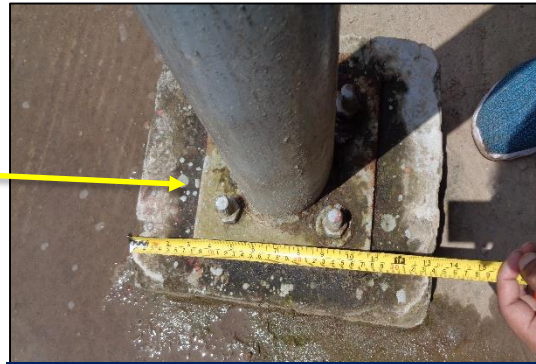
Short column measurement
