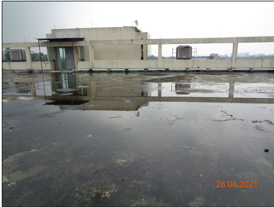
Water ponding at roof
