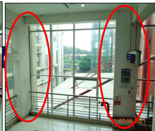
Orientation of marked column found mismatched
