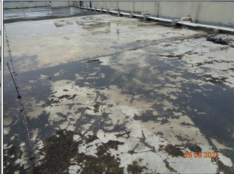
Water ponding at roof
