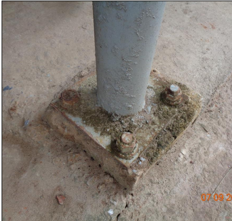
Corrosion in steel column
