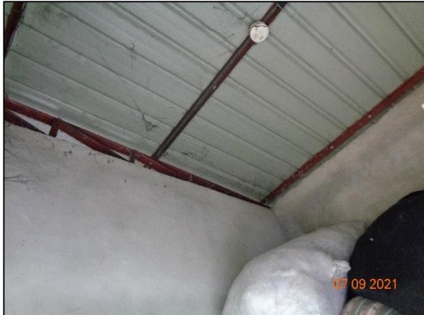
Truss roof System
