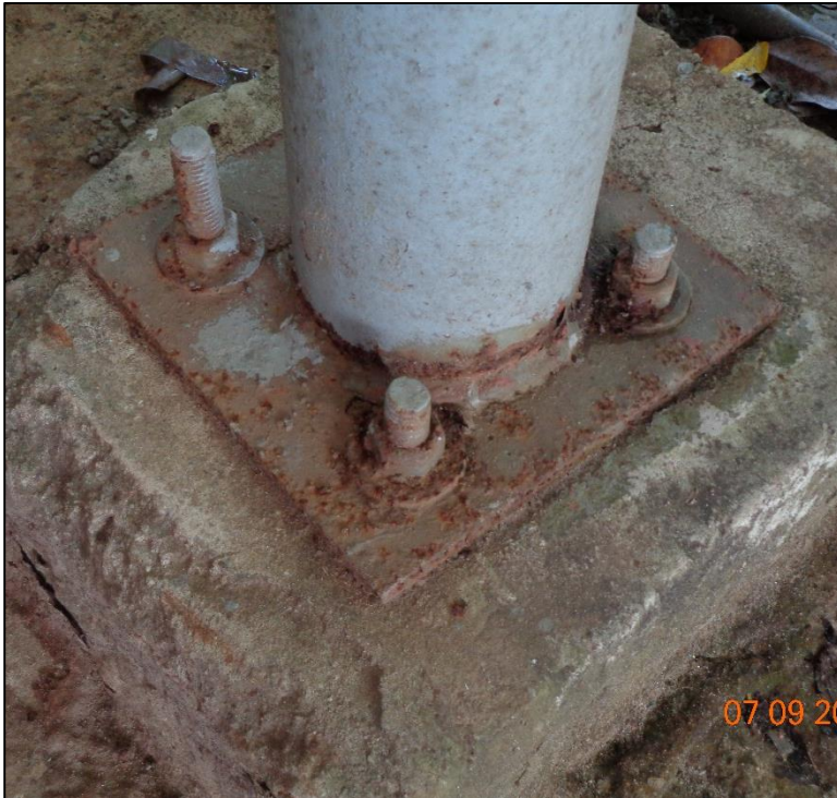
Corrosion in steel column
