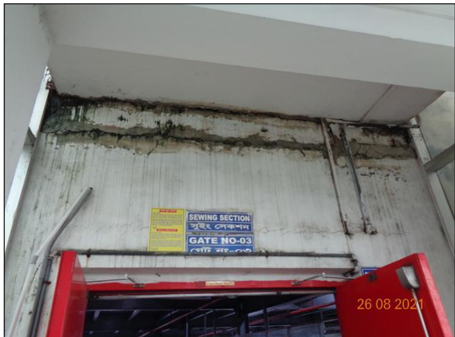
Dampness found in brick wall.
