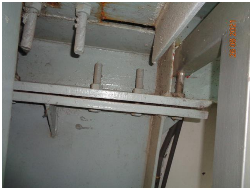
Gap observed in Beam- Column connection
