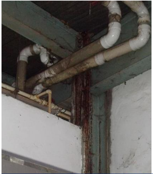
Corrosion in steel beam, column & beam-column connections
