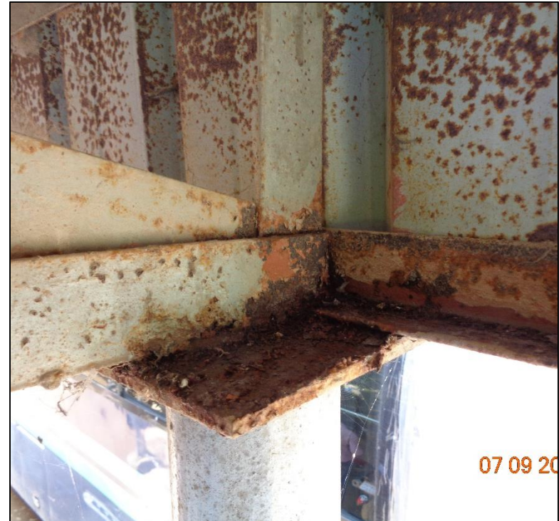
Corrosion in steel column
