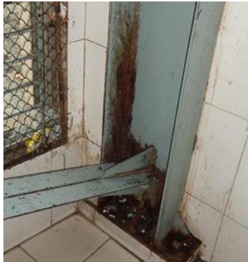
Bracing-Column Connection
