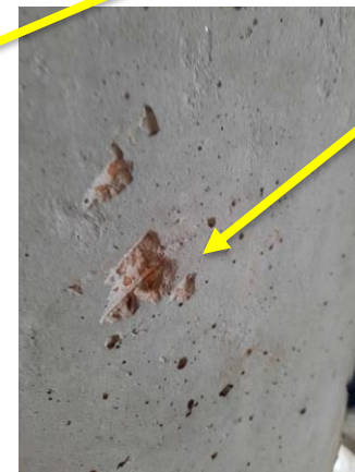
Brick aggregate [Generator Building]
