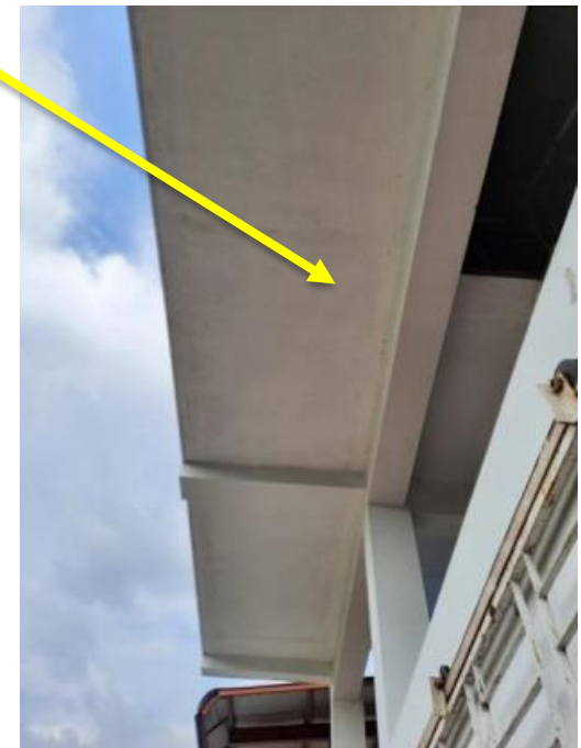
Cantilever Portion-Not Shown in Drawing
