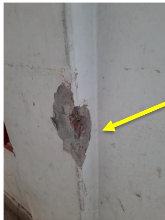
Brick aggregate [Main Building]
