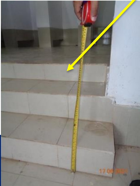
500 mm Buildup at 1 st Floor Toilet Block.
