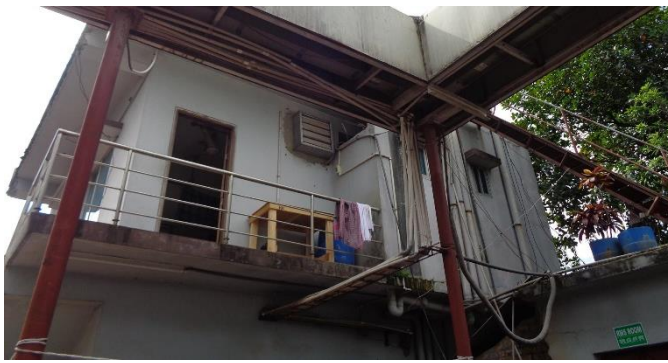
Toilet on the cantilever area
