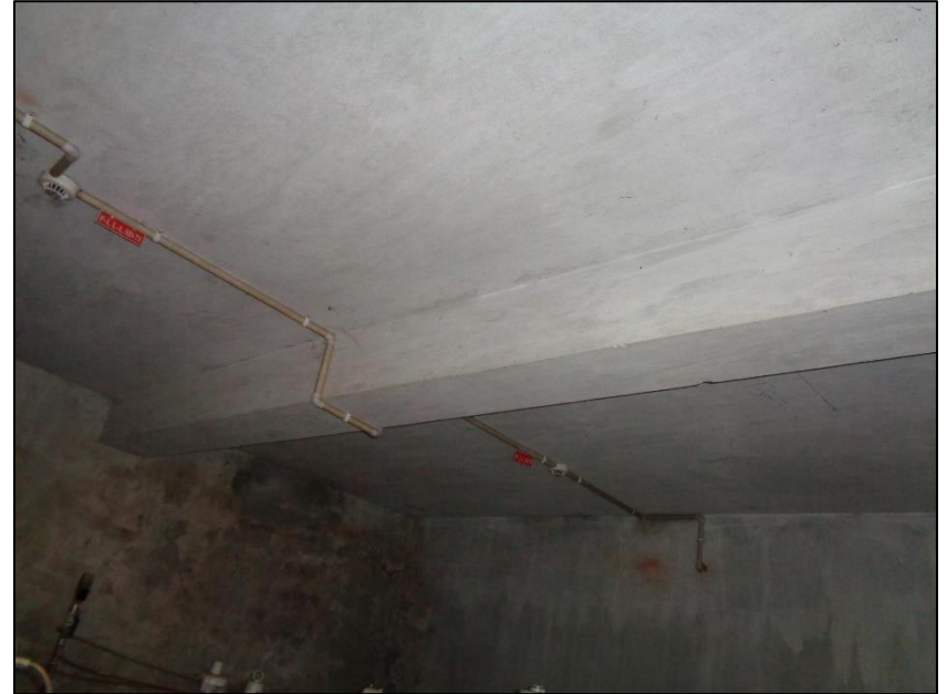
Interior of the building
