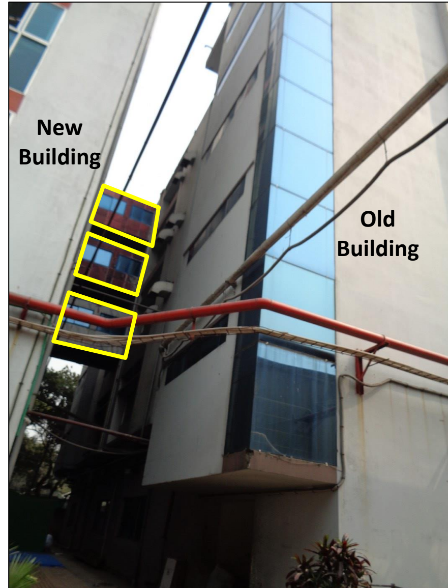
Connecting bridges at 2 nd , 3 rd & 4 th floor levels
