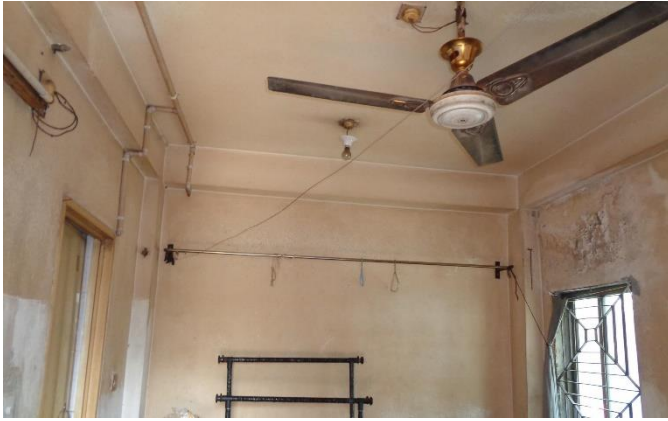
Interior of the building
