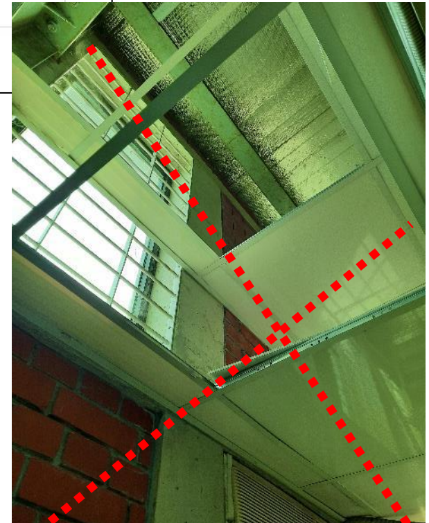
Missing Bracing
