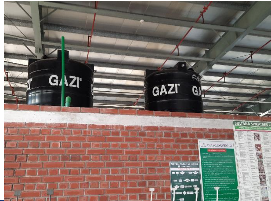
Water tanks are supported on the 125 mm and 250 mm brick walls. Building engineer is required to check the load carrying capacity of the walls.
