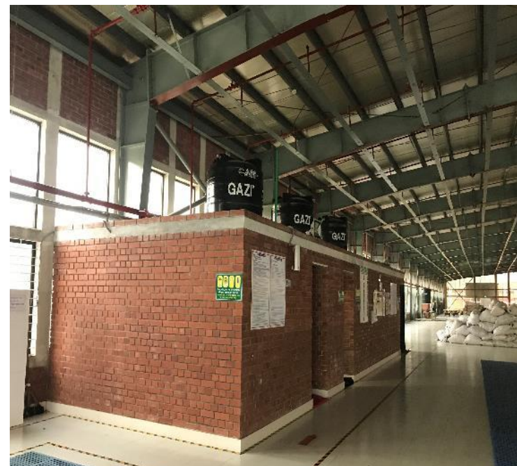
Bracings are interrupted in toilet zone (Shed 4,5,6,7)
