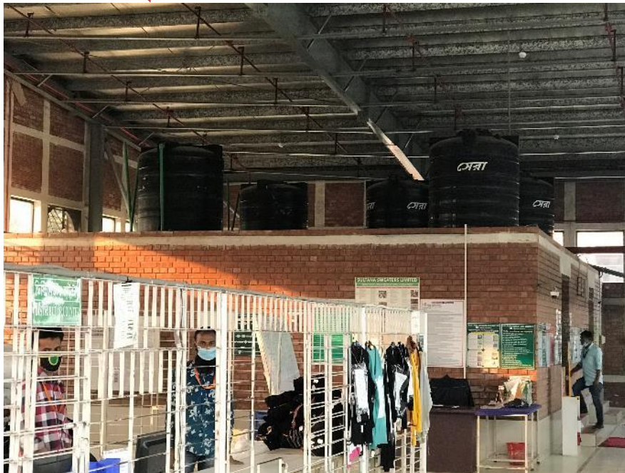
Water tanks are supported on the 125 mm and 250 mm brick walls. Building engineer is required to check the load carrying capacity of the walls.
