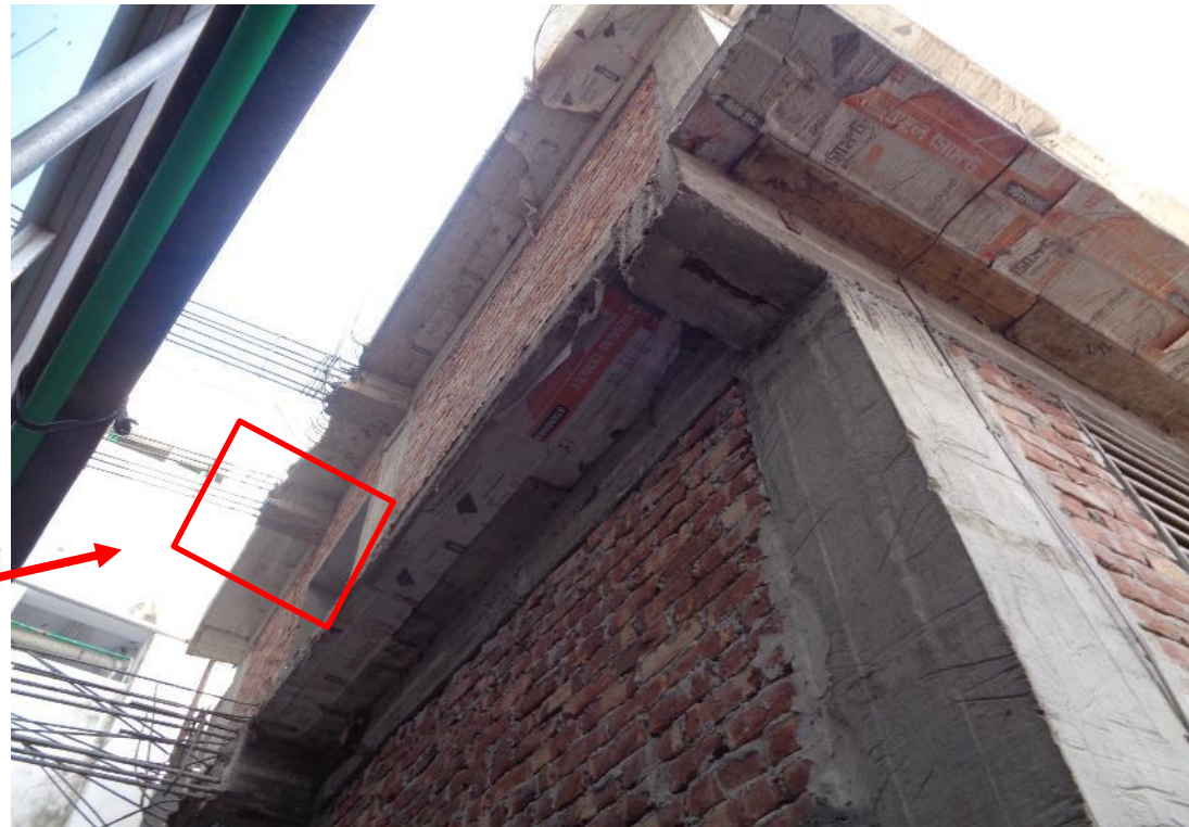
Extra beam at roof level
