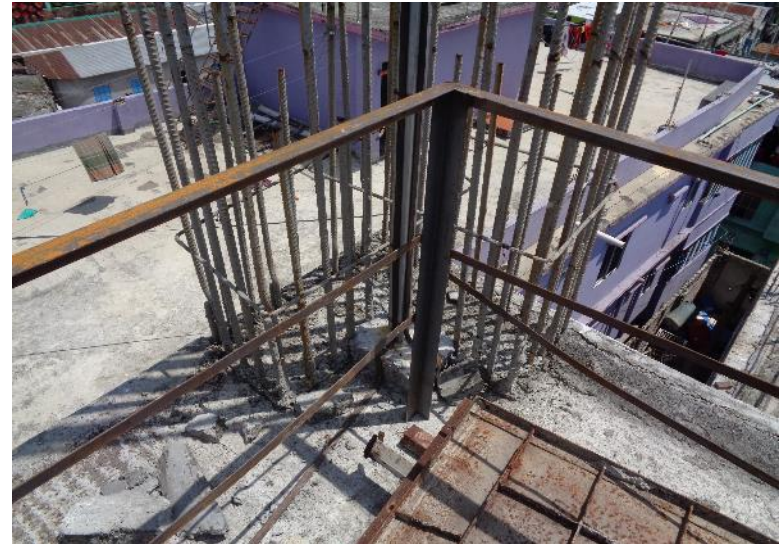
38-rebar at grid B1-9A
