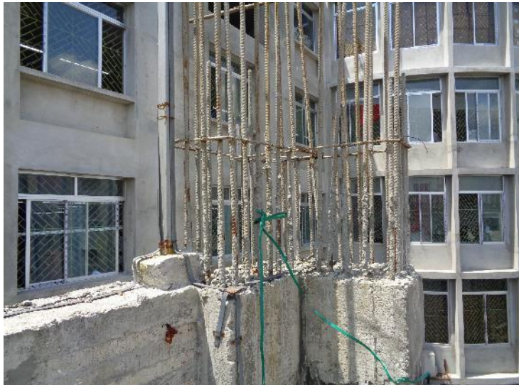
36-rebar at grid L-2
