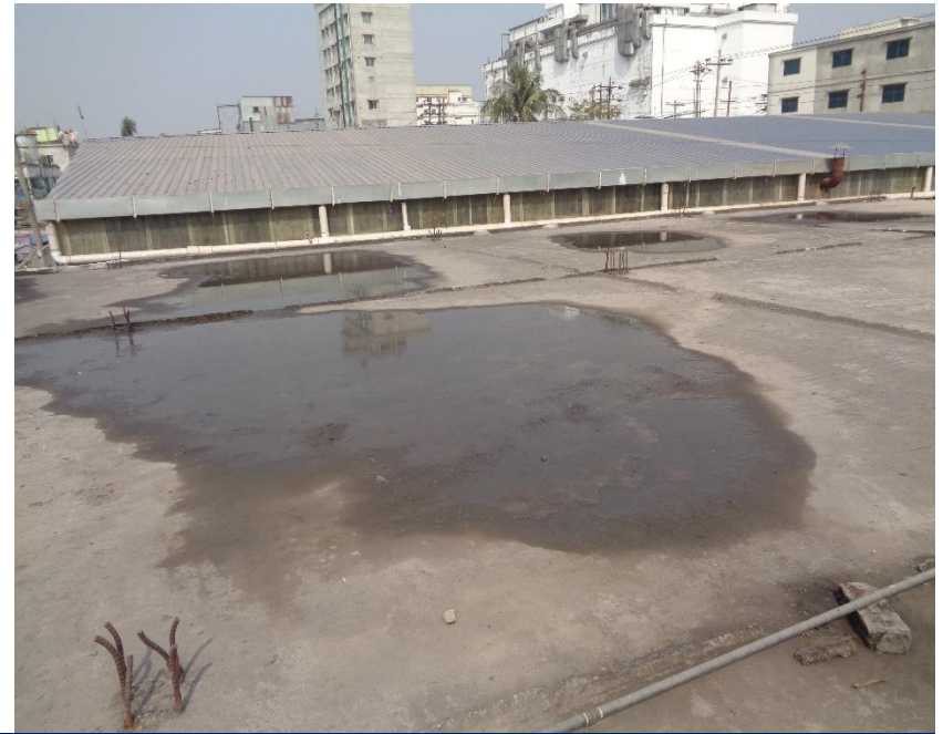
Water ponding on roof slab
