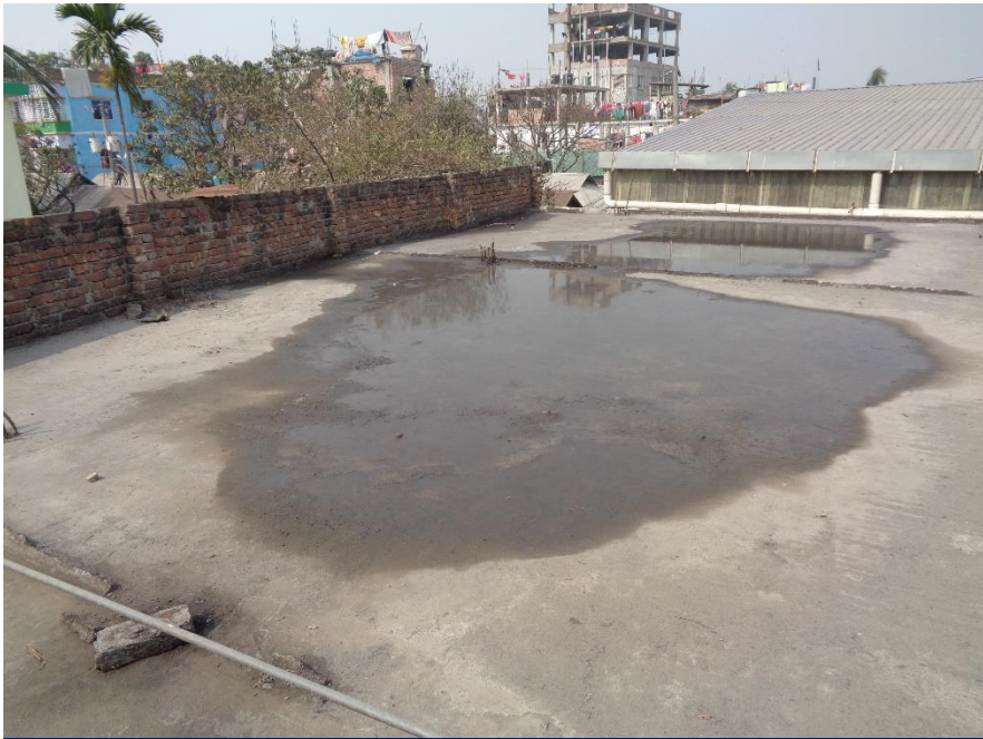
Water ponding on roof slab
