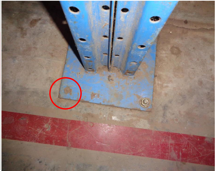
Missing bolts at support
