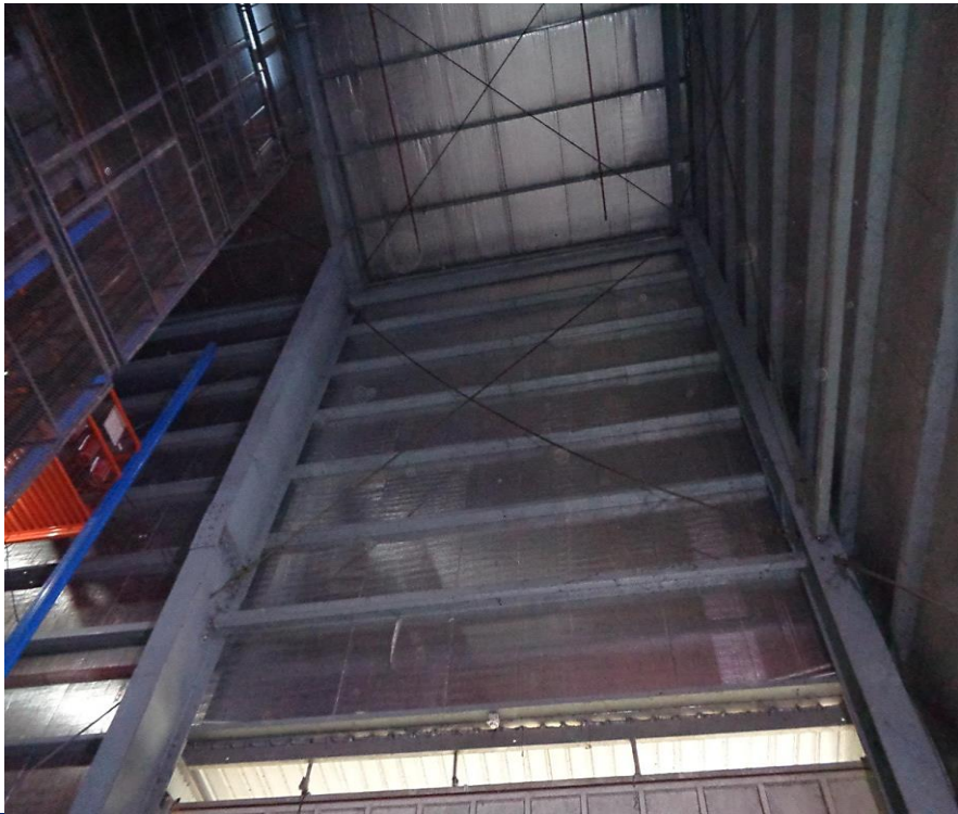
Loose cable bracing
