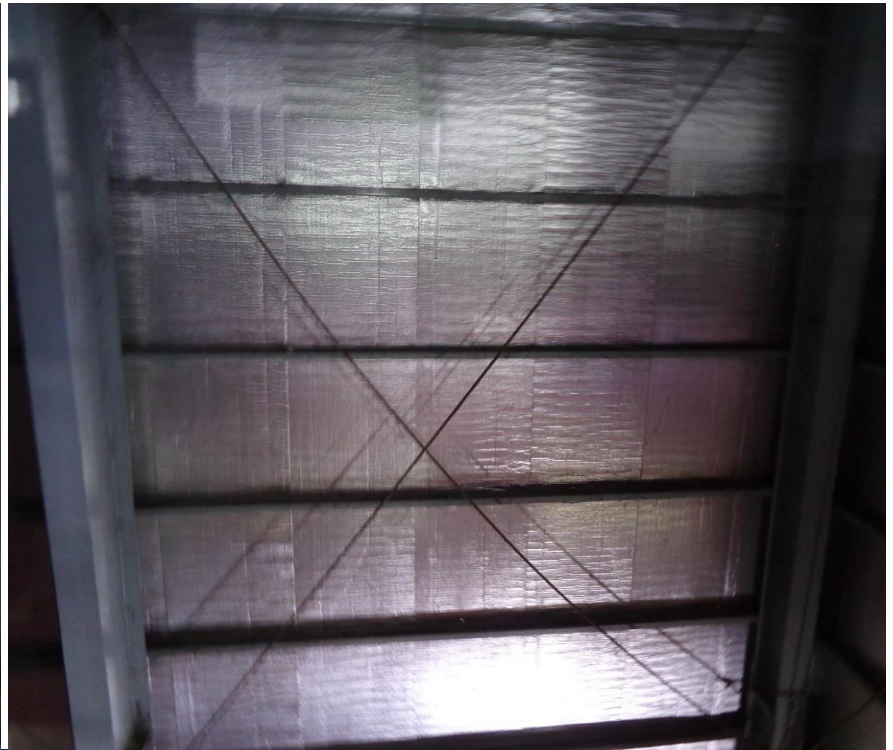
Loose cable bracing
