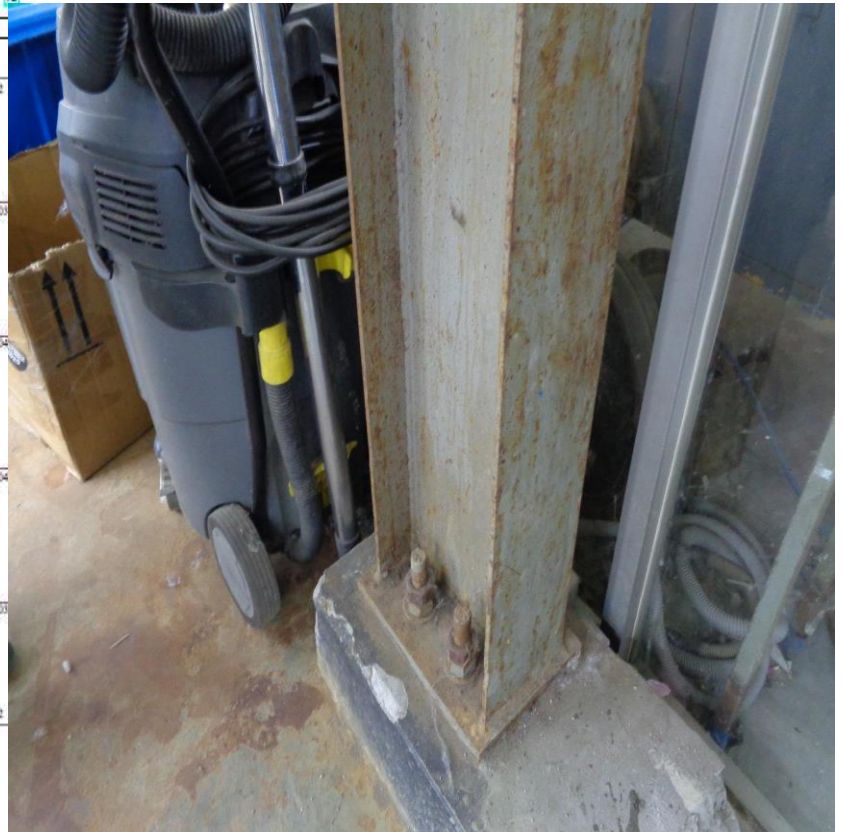
Corrosion in steel column
