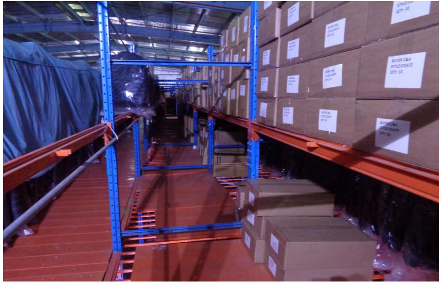
Storage load resting on multi storied steel rack
