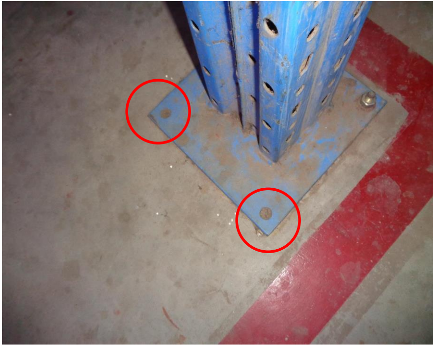
Missing bolts at support
