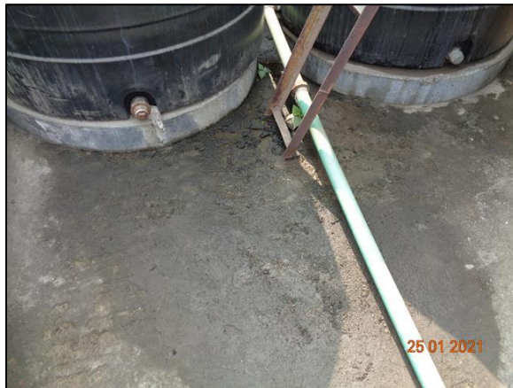
Dampness in roof top slab
