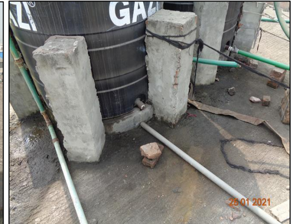
Dampness in roof top slab
