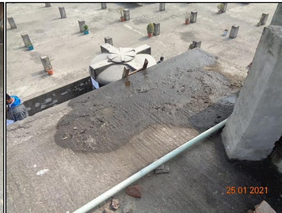
Dampness in roof top slab
