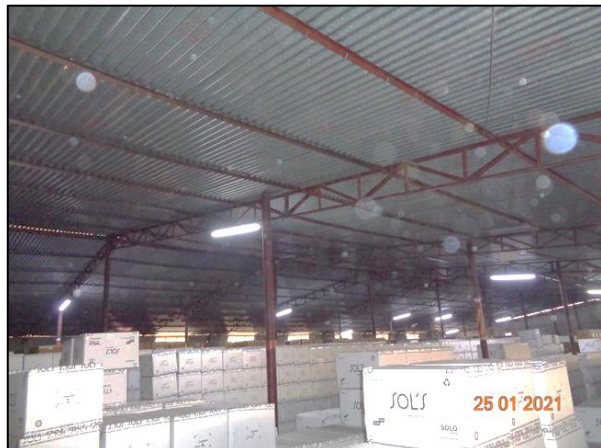
Truss roof System
