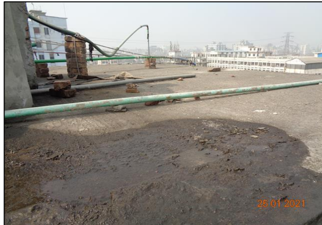
Dampness in roof top slab
