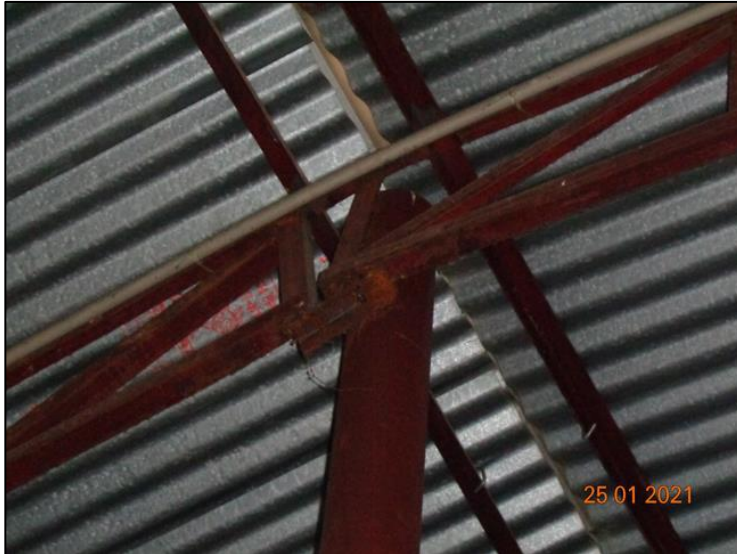
Corrosion in steel column
