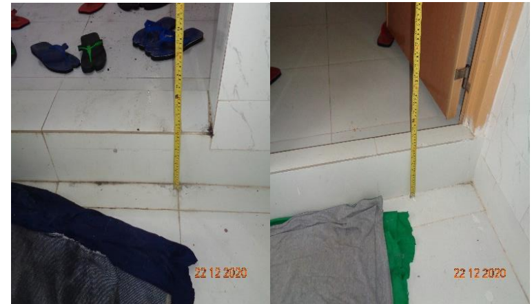
Build-up at toilet zone
