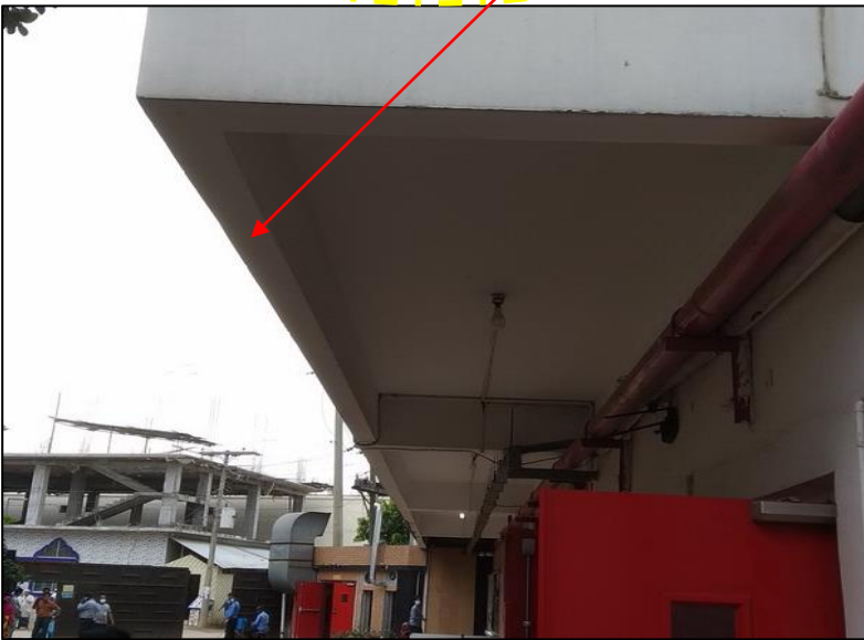
Edge beam on south side
