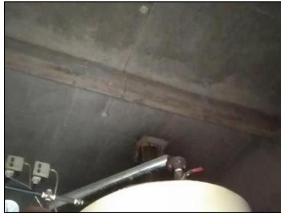
Beam on mid span
