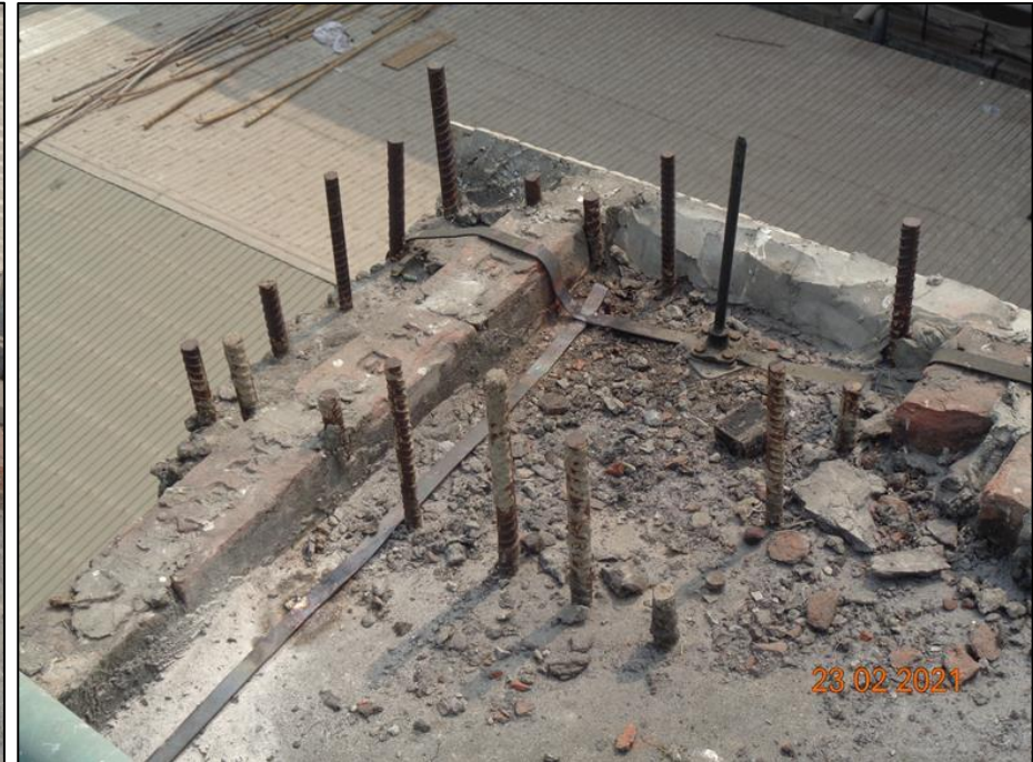
Exposed rebar at stair roof
