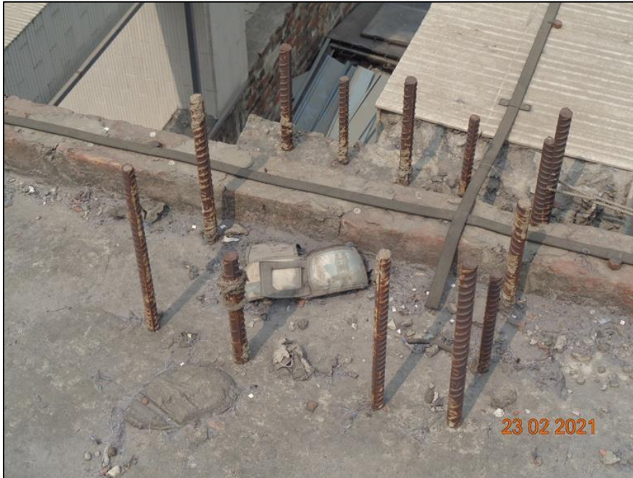
Exposed rebar at stair roof
