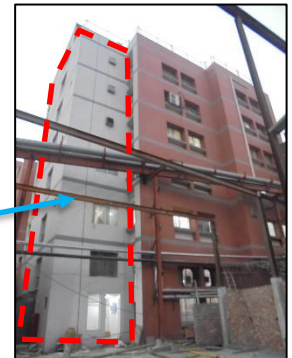
Cantilever toilet at south-east corner
