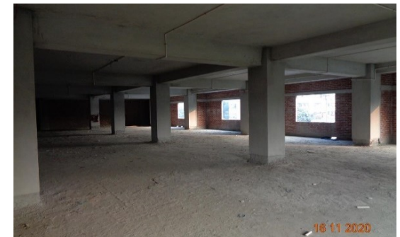
Inside Building 13 (Lab Building)
