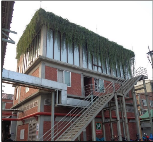
Building 10 (REB Building)
