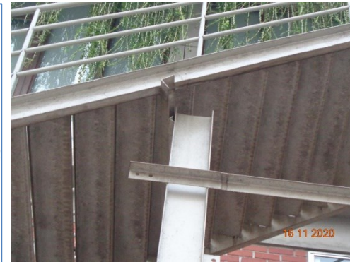
Column-rafter connection
