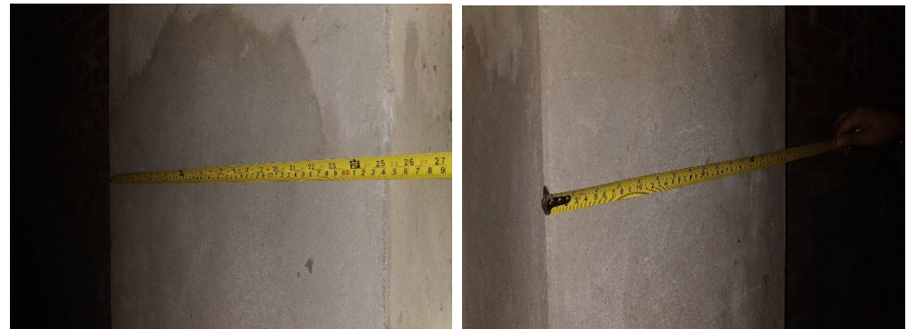
Column was measured to be 16" x 25"
