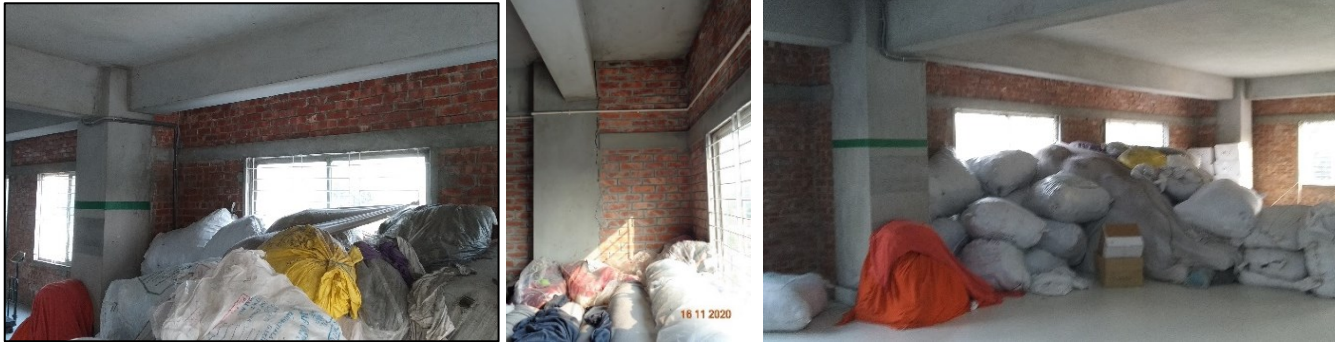
Loading in the cantilevered areas
