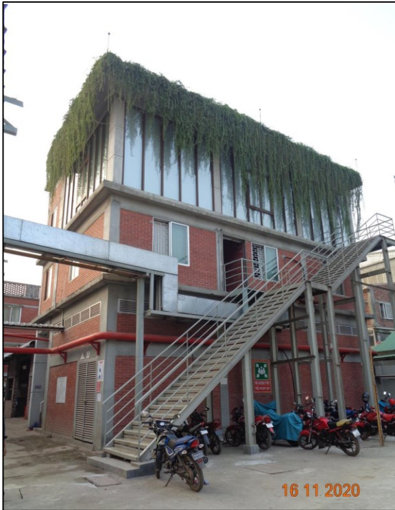
Inside Building 10 (REB Building)
