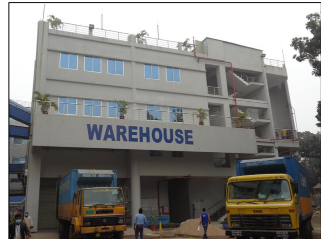
Building constructed up-to two storied
