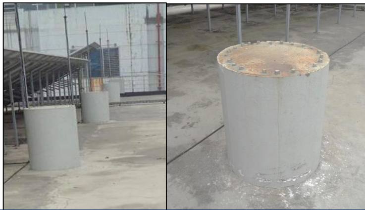
Extended column re-bar at roof/2 nd floor
