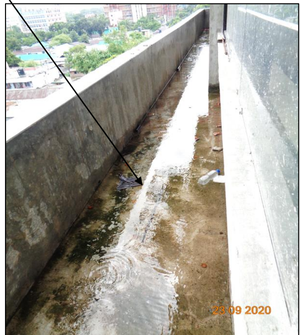
Water ponding at 3 rd floor cantilever
