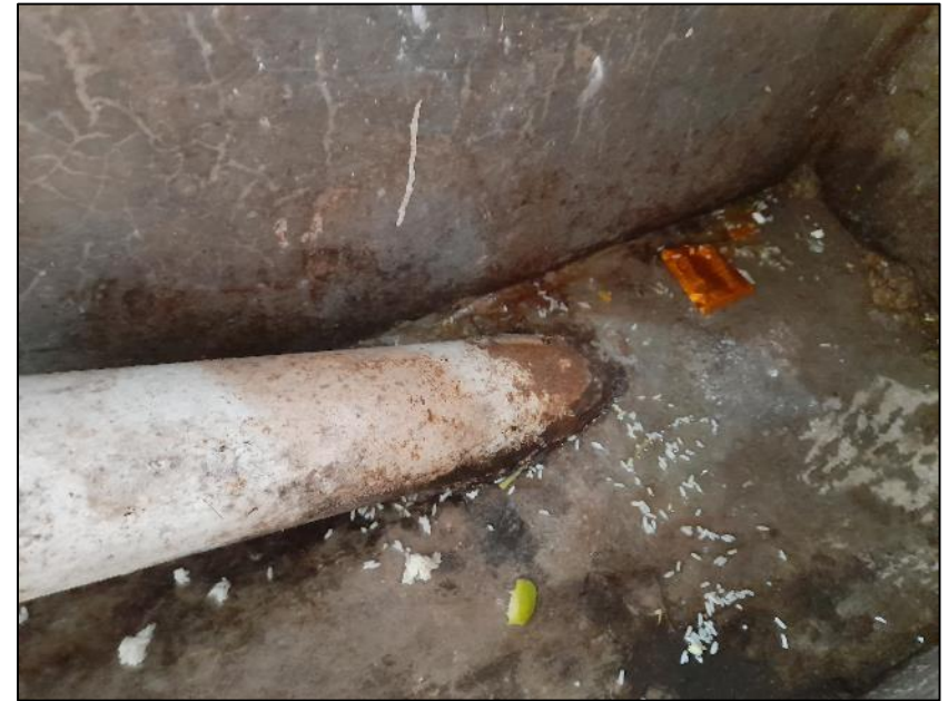
Signage of corrosion observed at vertical bracing
