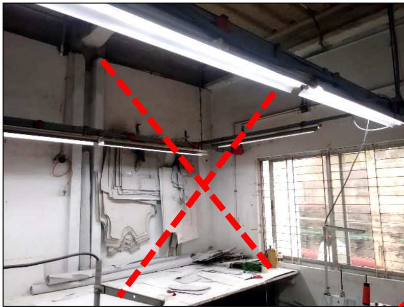
Vertical bracing found missing
