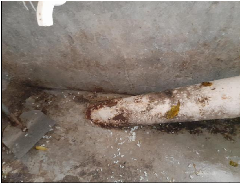
Signage of corrosion observed at vertical bracing
