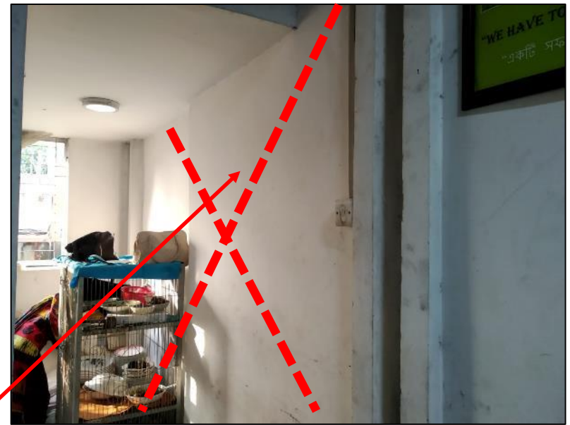
Vertical bracing found missing
