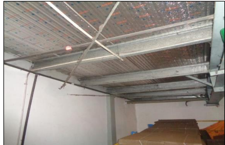
Inactive cable bracing (inserted in partition brick wall)
