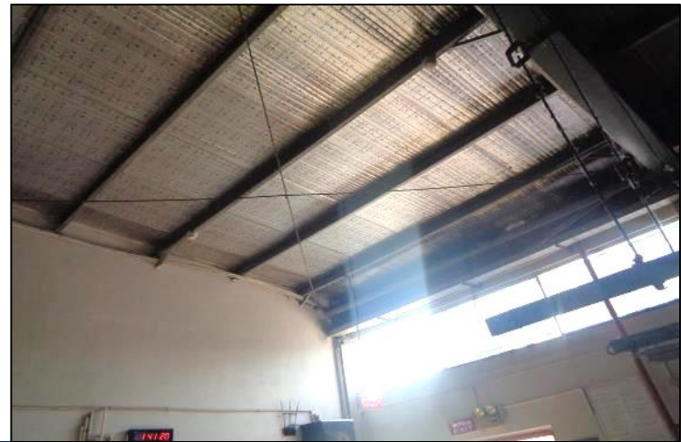
Loose cable bracing at several location
