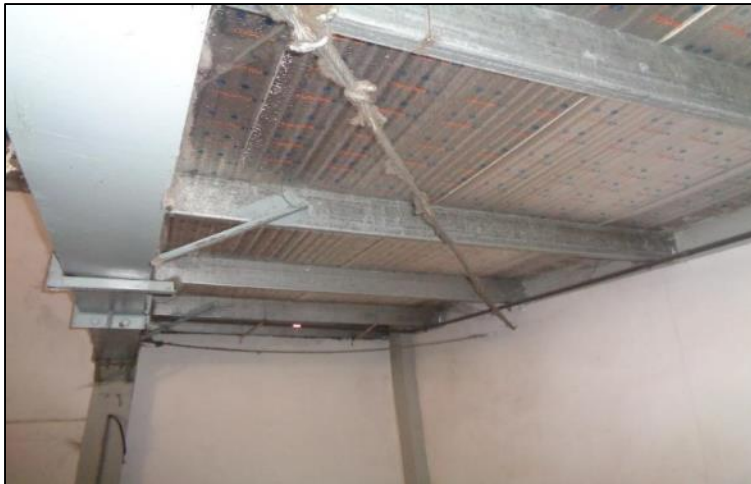
Inactive cable bracing (inserted in partition brick wall)
