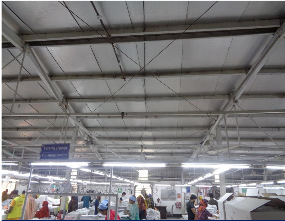
Loose roof bracing
