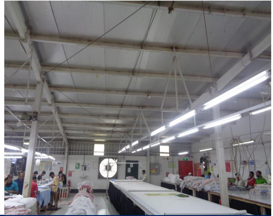
Loose roof bracing
