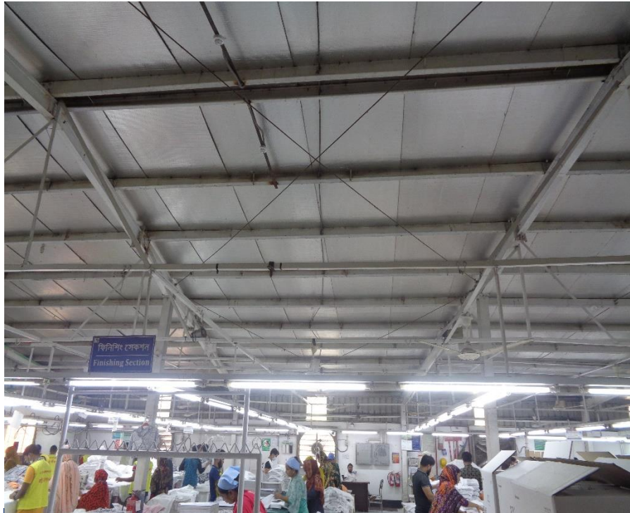
Roof bracing provided only
