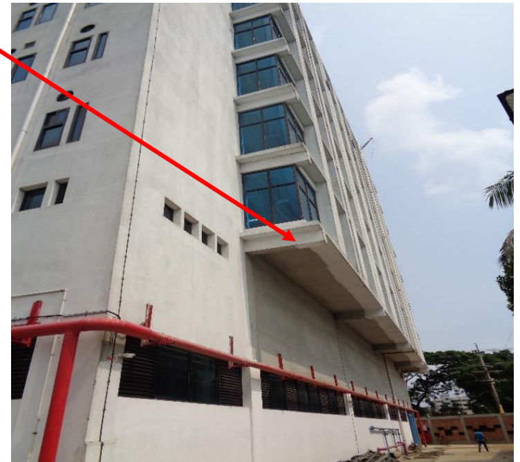
Cantilever at south side
