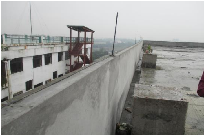
RC parapet on the roof
