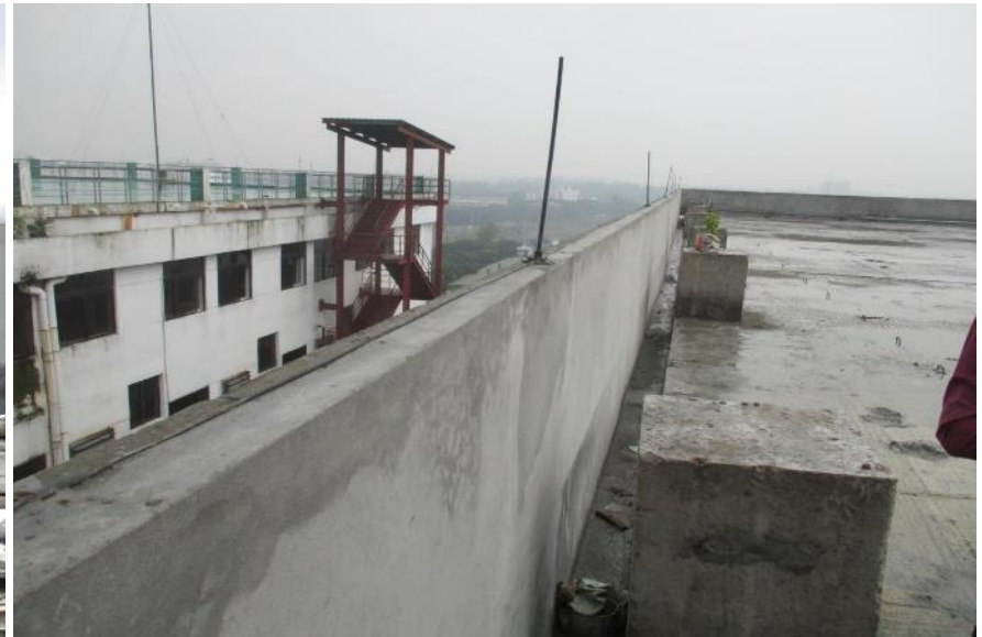
Free standing wall observed on the beam bottom cantilever slab.
