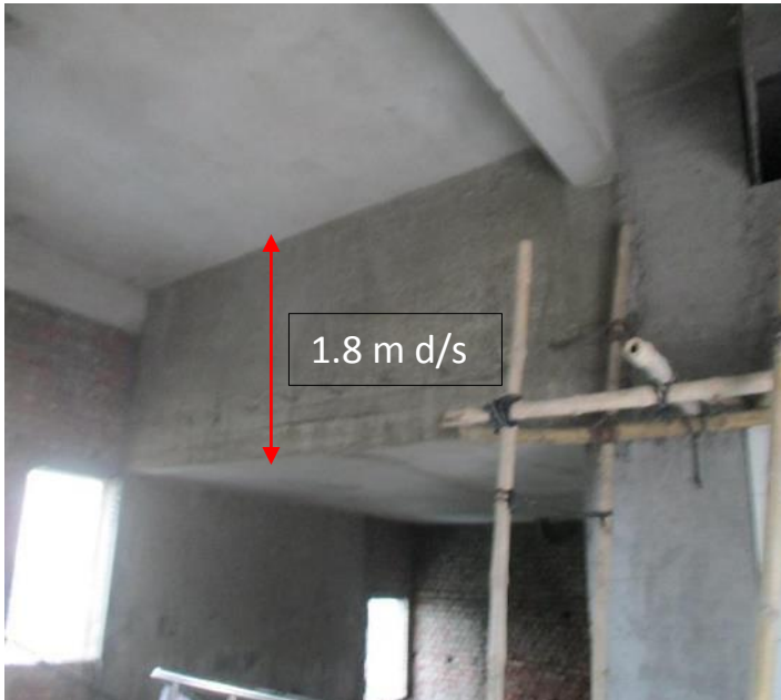
OHWT on the roof
