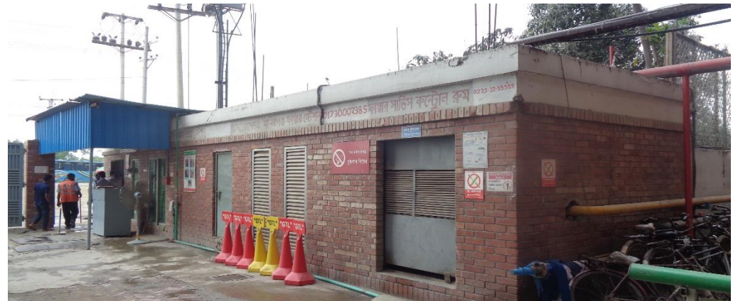
Gate House & RMS Room
