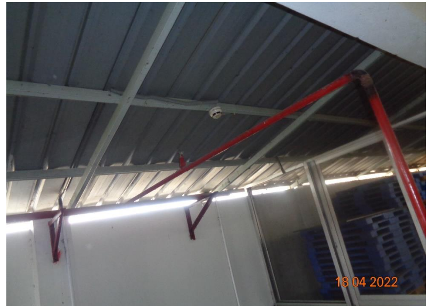
Lightweight roof of pump house
