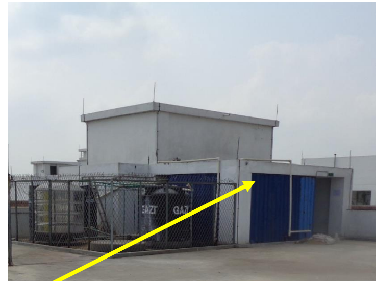
Additional room in front of stair
