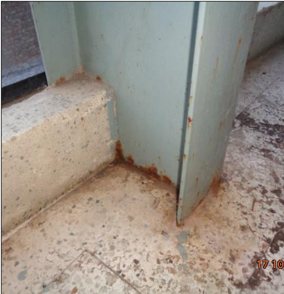
Corrosion was found in steel column
