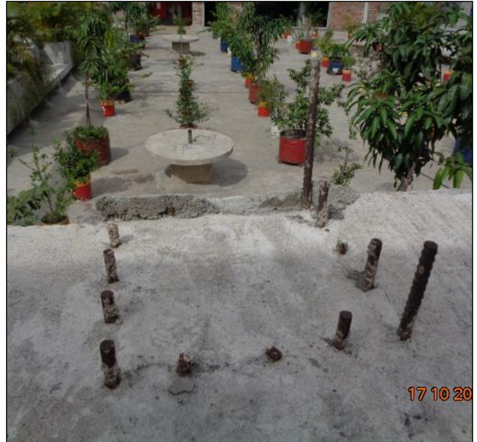
Exposed rebar at roof
