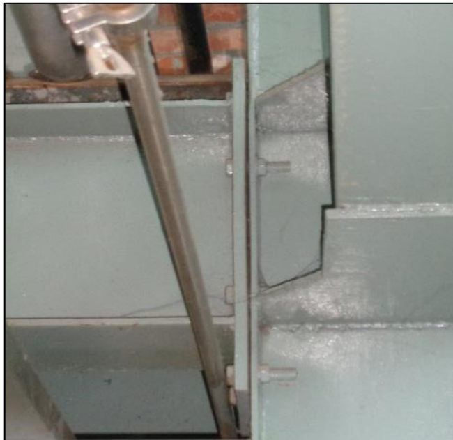
Connection gap was found in rafter-column connection
