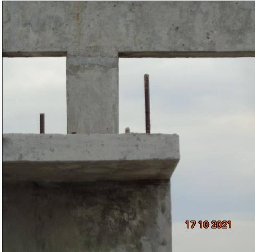
Exposed rebar at roof
