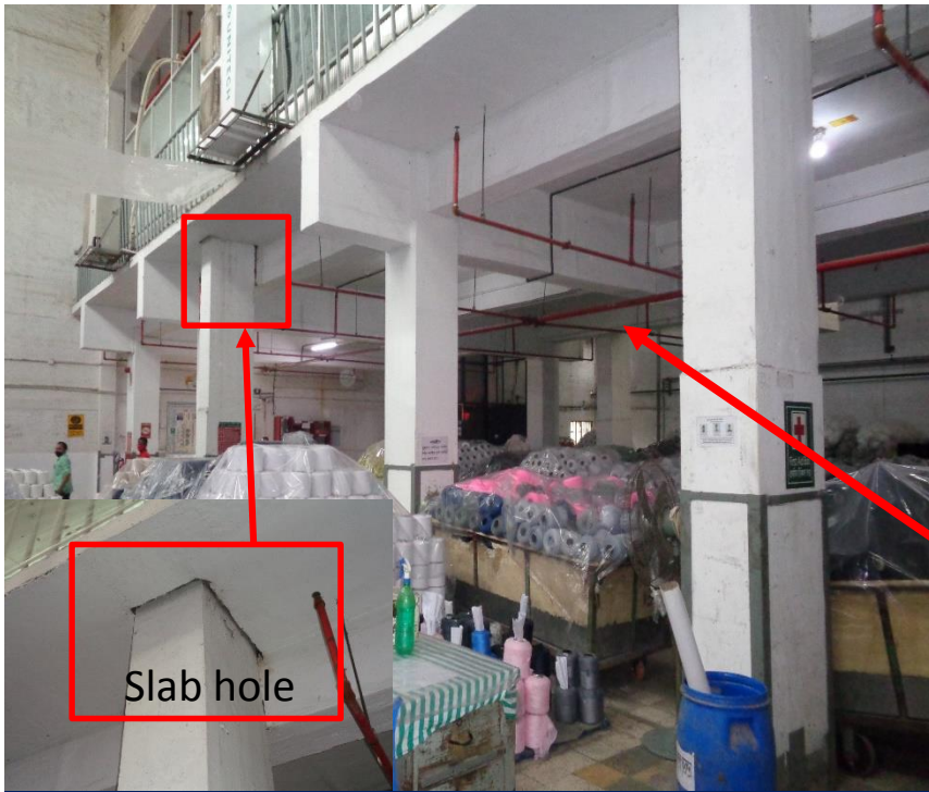
Rectangular hole in the slab not shown in the drawing
