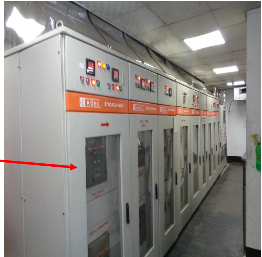
Columns not found on-site
