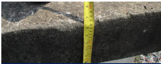
150 mm roof slab
