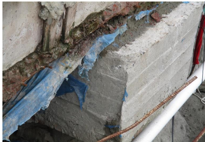
B-11: Stone aggregate on foundation
