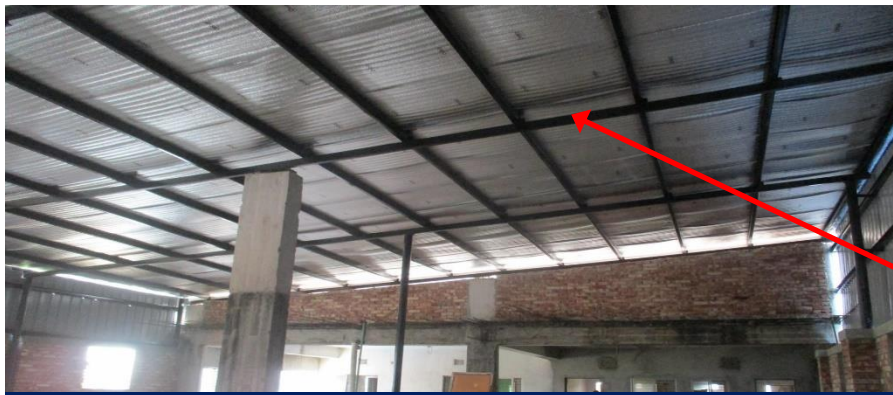
1st floor: Steel rafter on steel pipe & RC column
