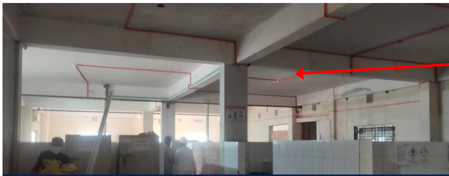
Ground & 1st floor: RC beam-column frame
