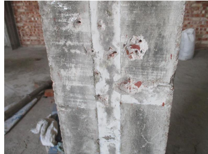
B-8: Brick aggregate on column
