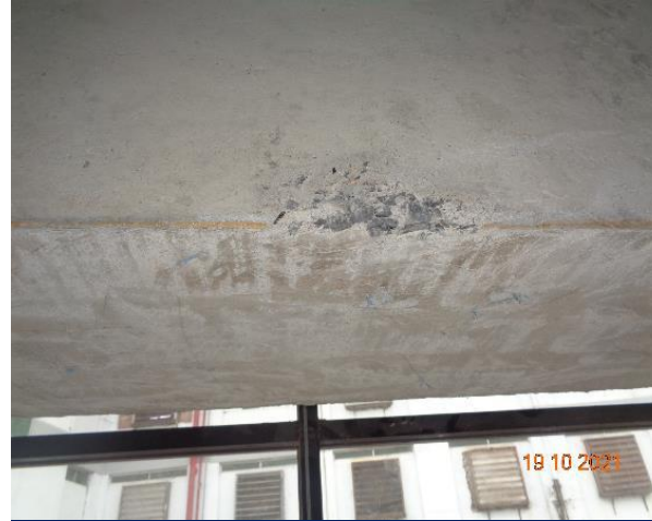
B-9: Stone aggregate on column and floor
