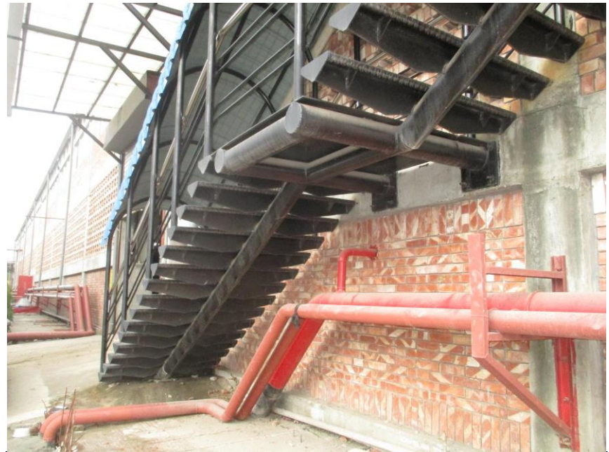
Design review steel stair is required
