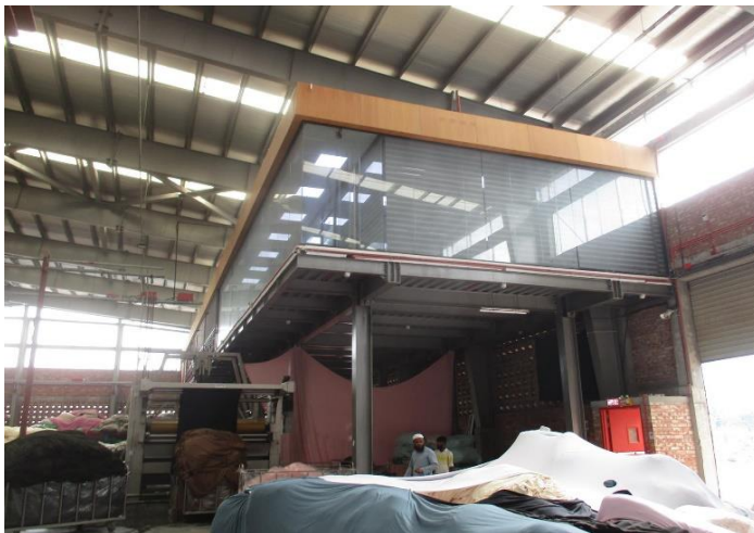
Design review required for mezzanine
