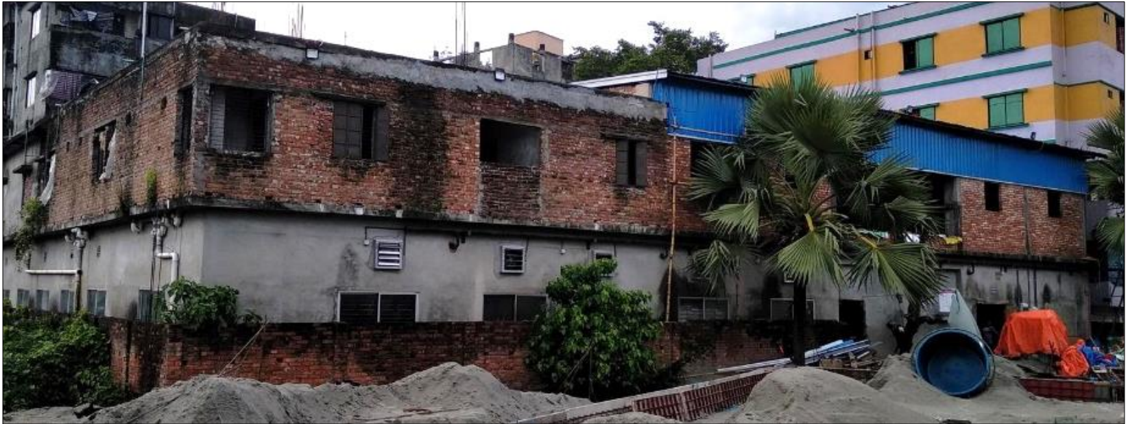
Geotechnical investigation report not available for Building- 8
