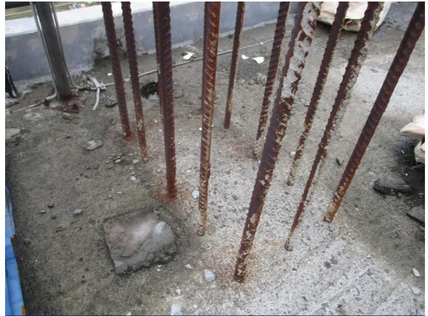
Rebar corrosion
