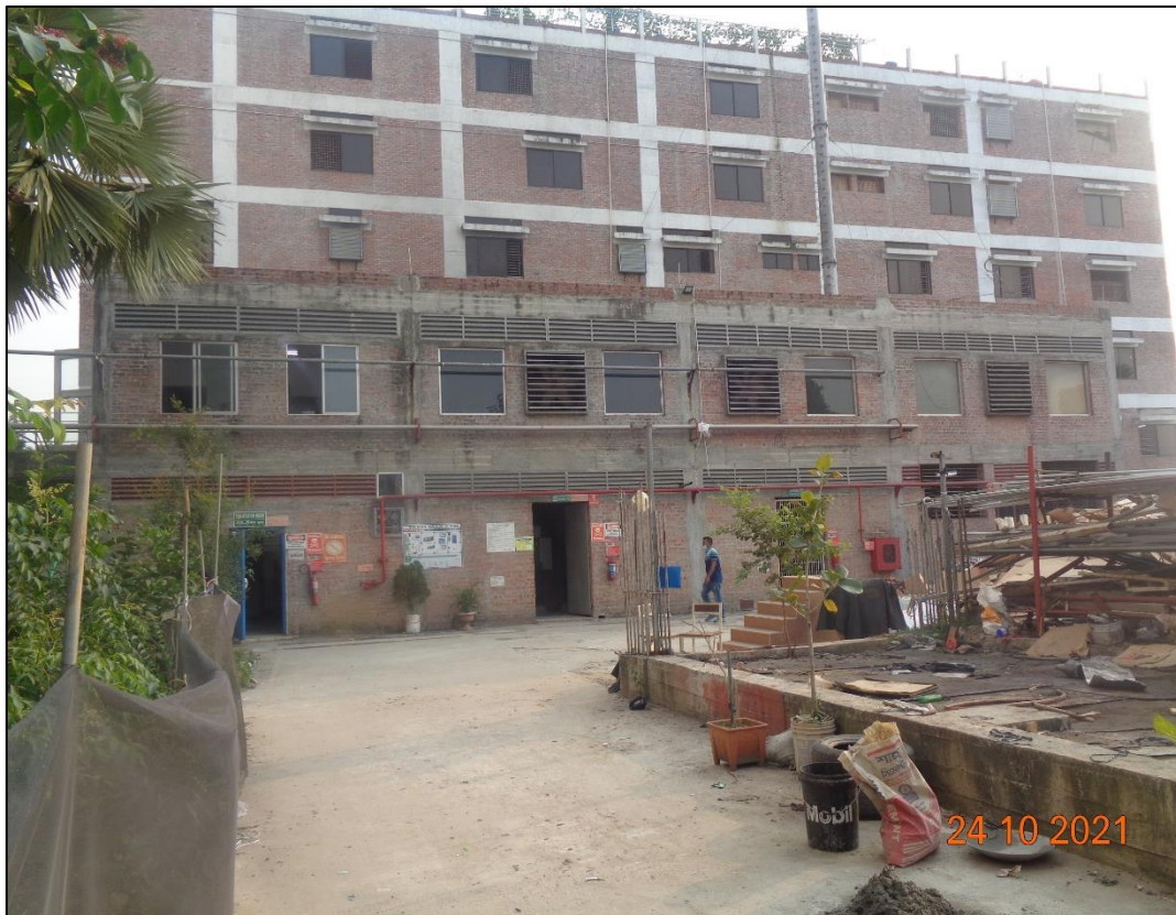
No design report for utility building
