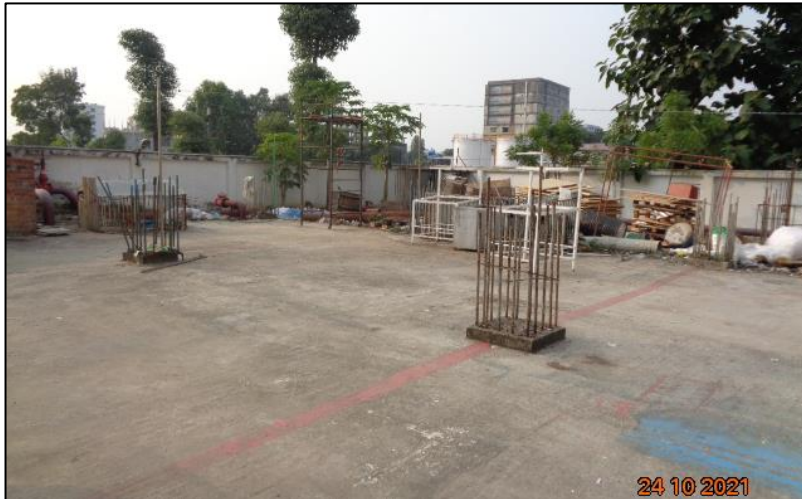
Extended column re-bar at ground floor
