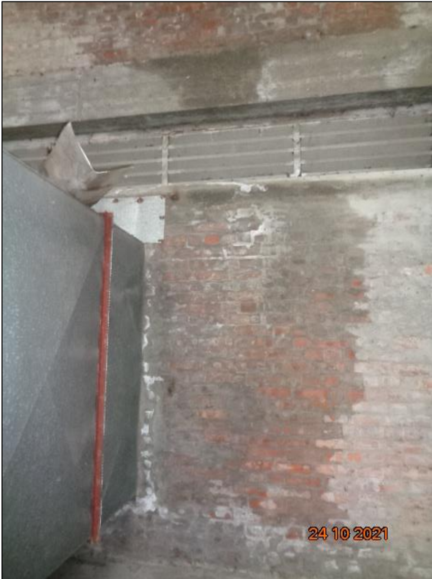
Dampness on brick wall
