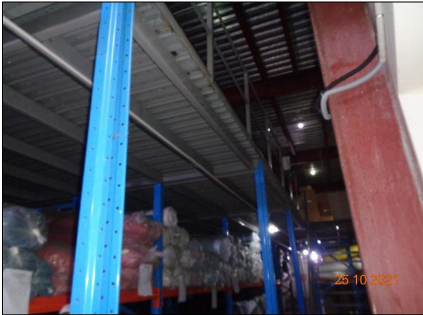
Mezzanine supported by rack post - Building 3
