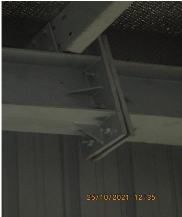
Connection gap – Building 4
