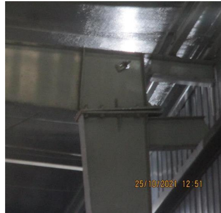
Connection gap – Building 5
