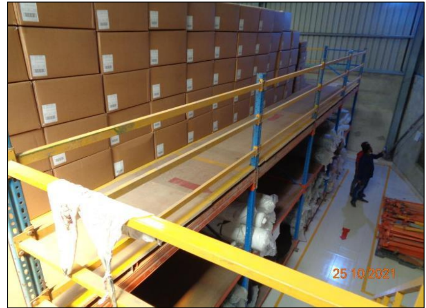
Mezzanine supported by rack post - Building 4
