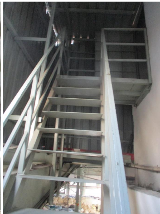
Steel stair connected with lift core brick wall
