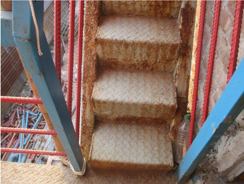
Loose cable bracing
