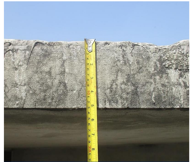
125 mm thick RC slab
