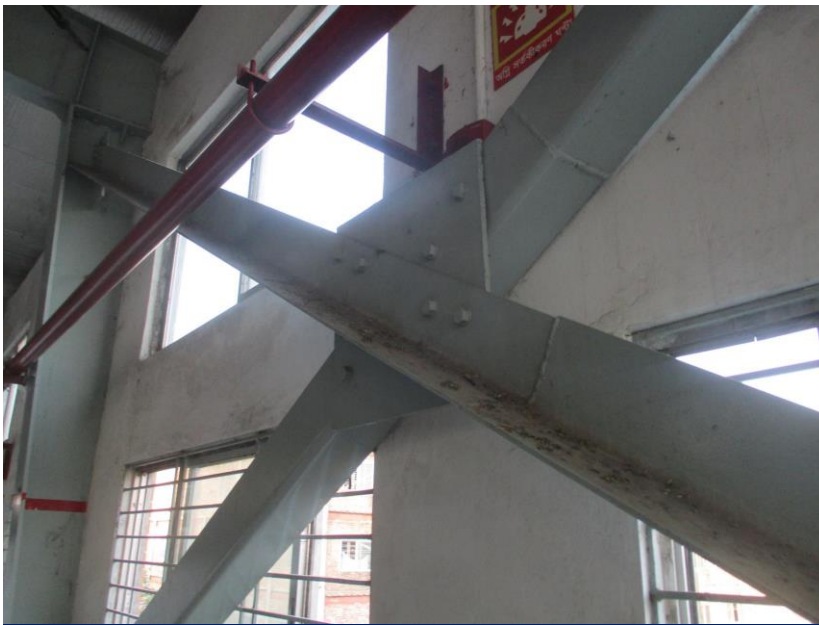
Vertical angle bracing on-site
