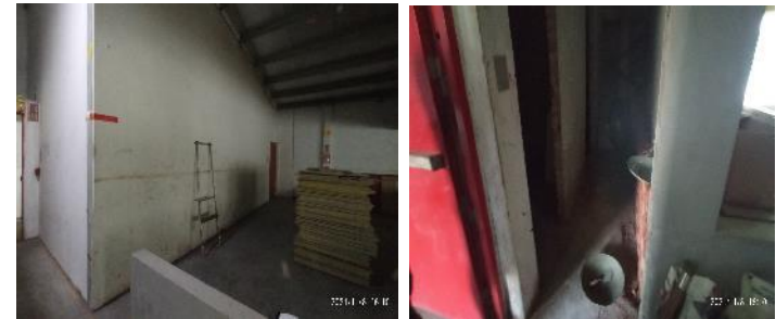
New toilet beside south side stair & shifting wall at storage
