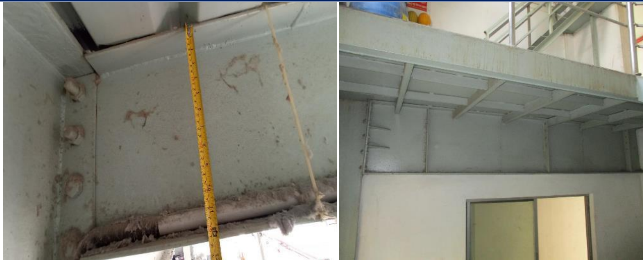
Miss match in beam (Web of SB1 found 310mm instead on 320mm & No extra plate was found in RMB1)
