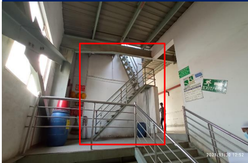
Steel stair at 1 st floor
