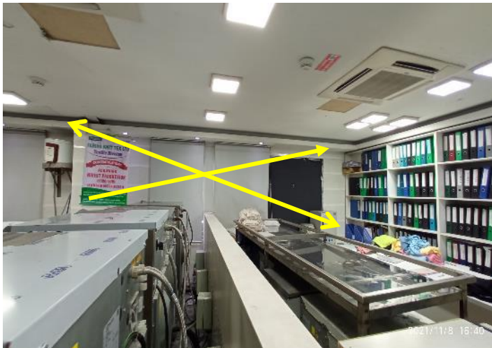
Missing bracing at different place
