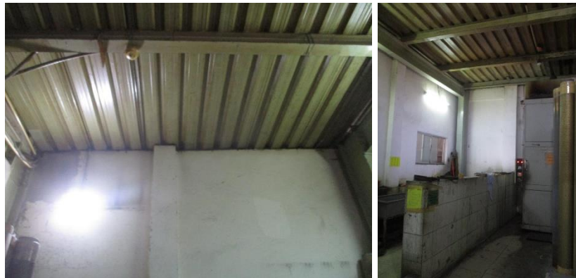
Expansion of mezzanine floor
