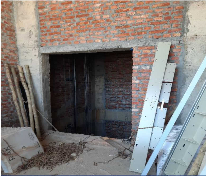
No guardrails around the lift core
