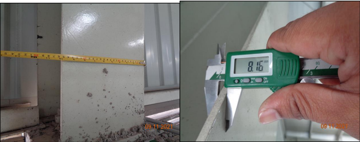
Size measured – Flange width: 250mm & Flange Thickness: 8mm
