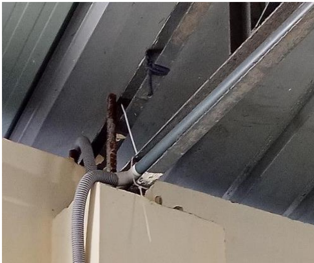
Truss welded with rebar of column
