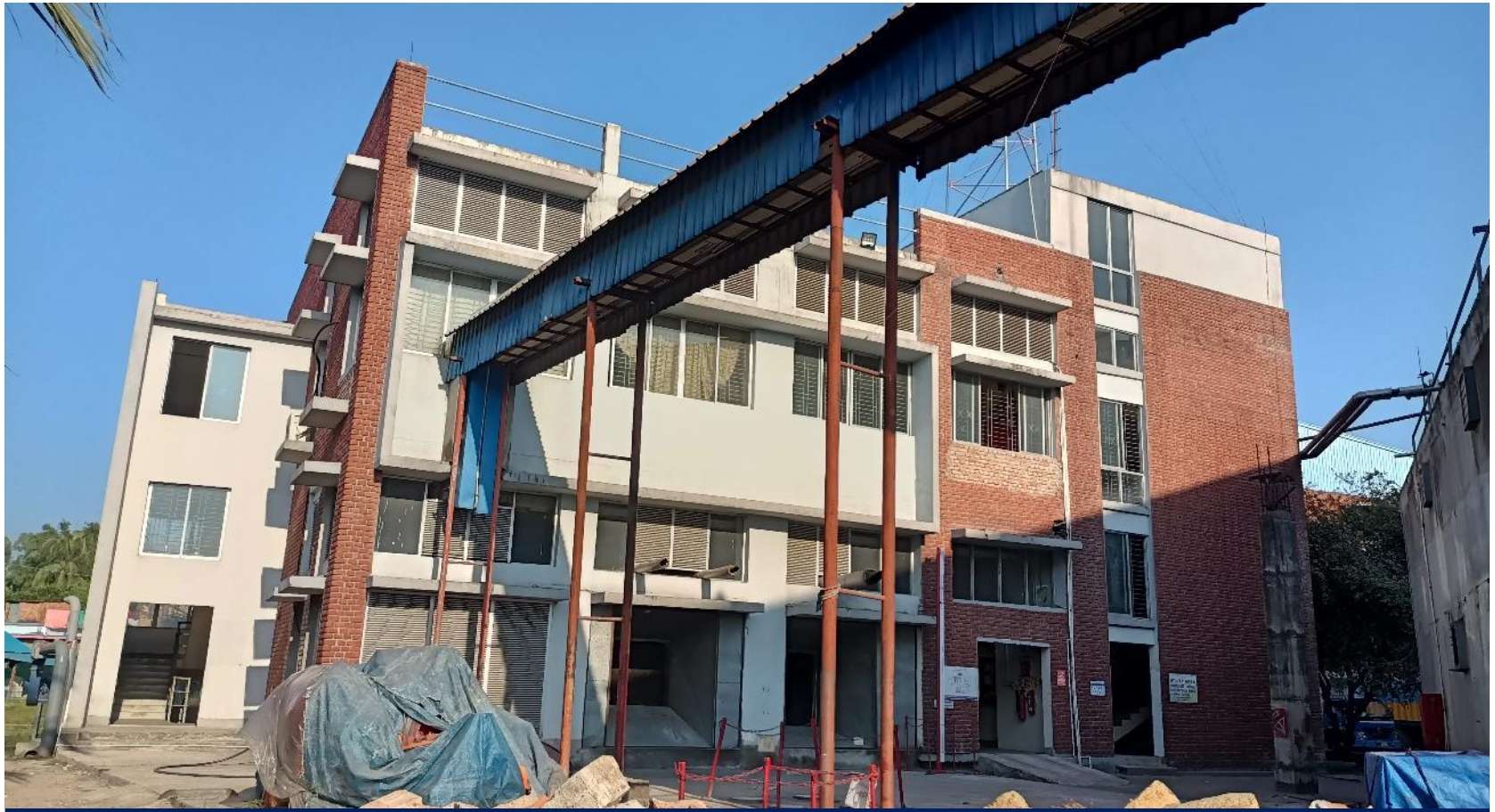
Two storied Utility Building
