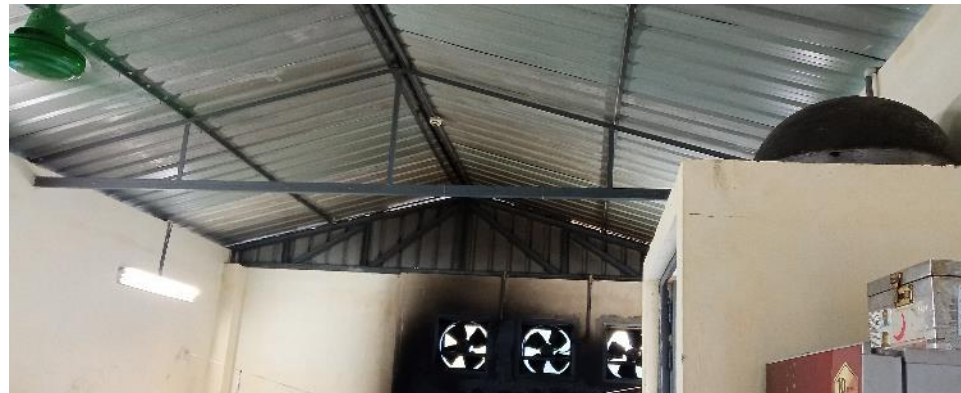
Truss section in as-built condition
