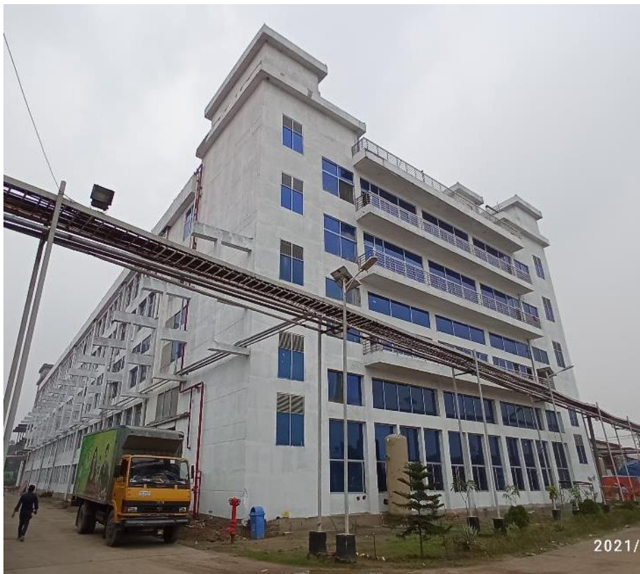
Building 4 (Production Building)
