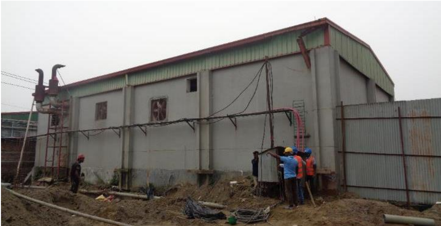
Building-2 (Substation Shed)
