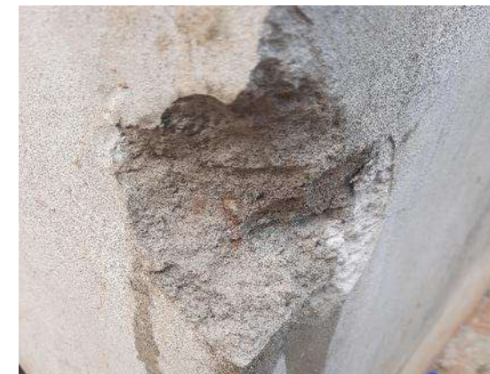
Stone aggregate (Security Building)
