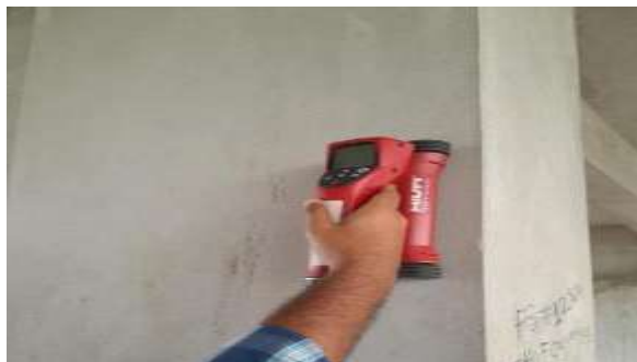
Rebar scan to confirm rebar quantity
