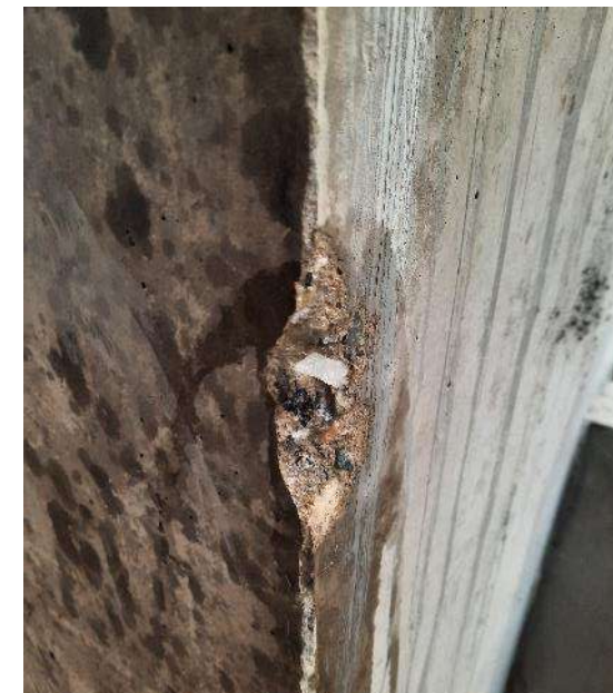
Stone aggregate (Utility Building)
