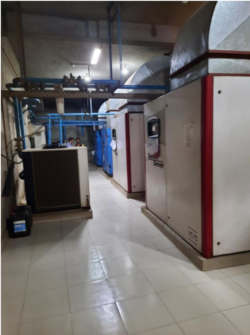
Generator machine at 1 st floor of Utility Building
