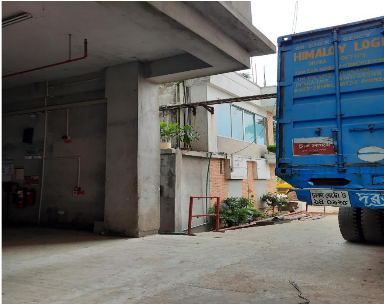
Ground Floor Column at Parking
