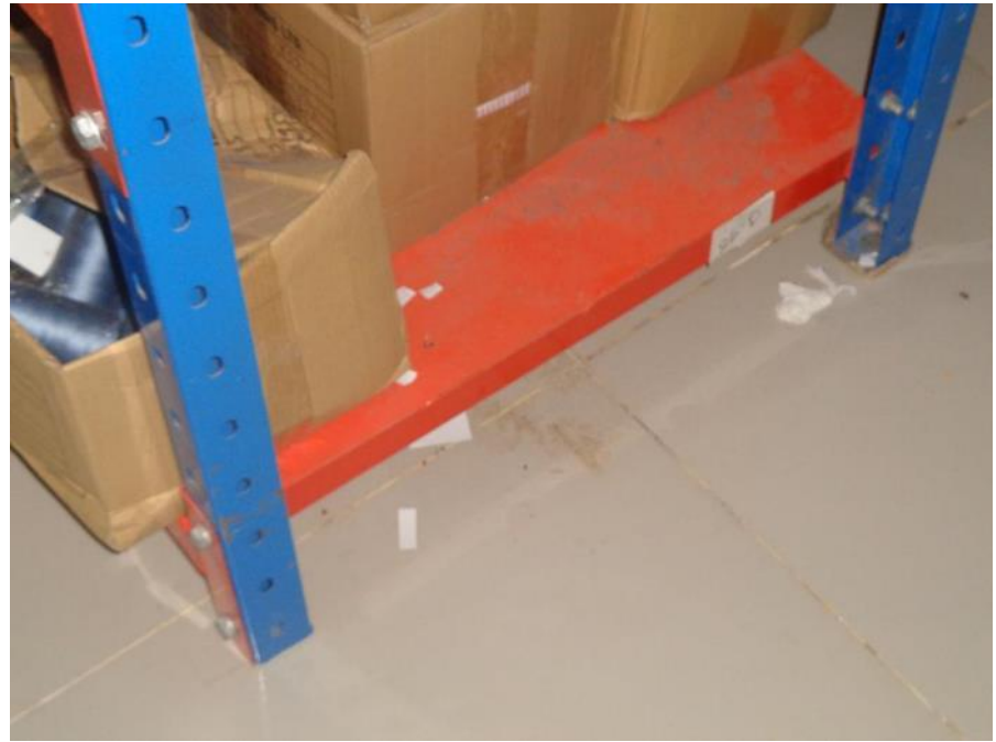
Storage rack without bracing and not anchored
