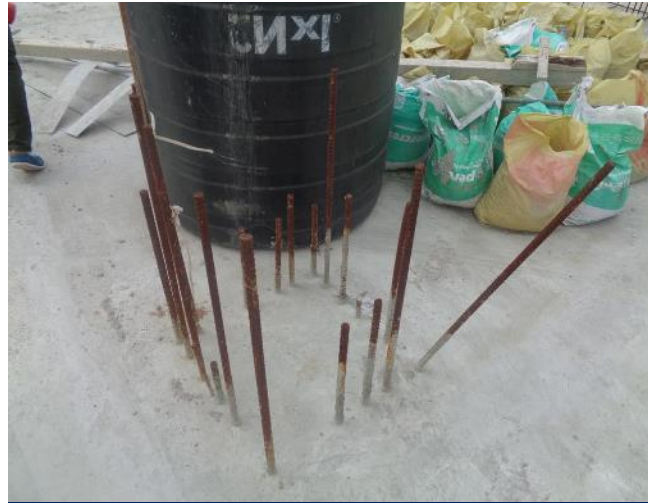
Exposed rebar
