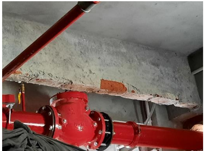
Unrestrained brick wall at stair without lintel/support.
