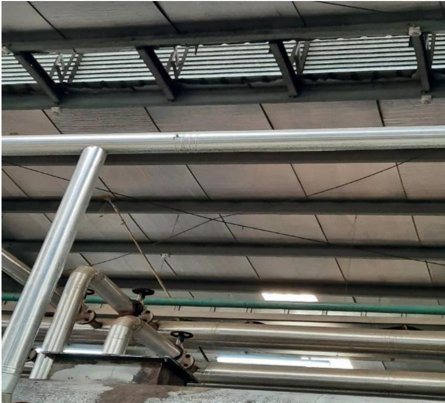
Loose and inactive cable bracing
