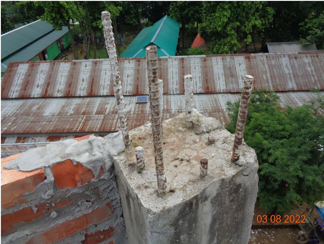
Exposed rebar at roof
