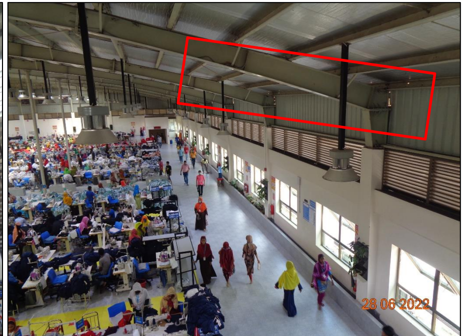
Steel roof shed - Lateral load transfer media missing at roof level
