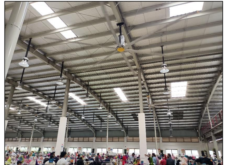
Steel roof shed - Lateral load transfer media missing at roof level
