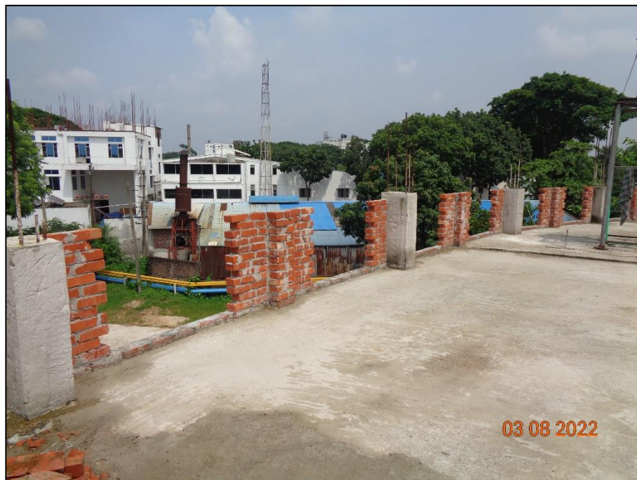
Parapet wall missing at roof
