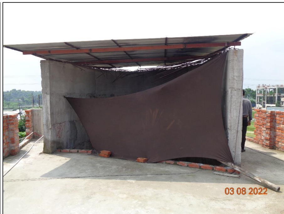
Parapet wall missing at roof
