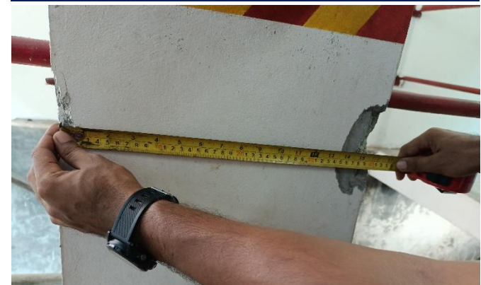
C-03 column 375 mm instead of 400 mm
