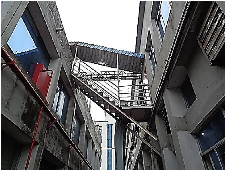
Connecting stair between the production building & head office building.
