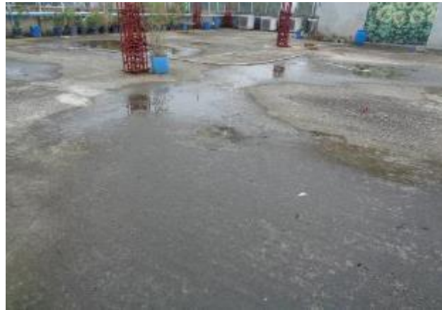
Water clogging on the roof and dampness on wall & beam
