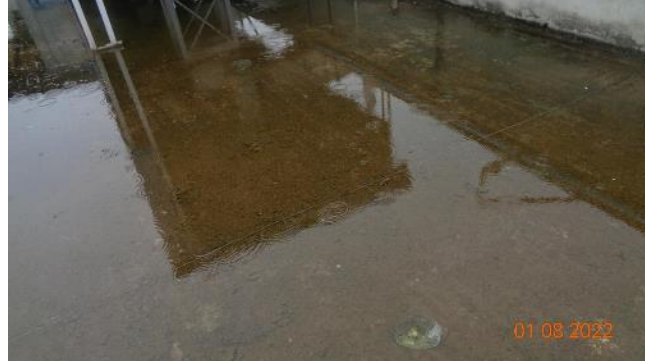
Water clogging on roof.
