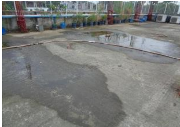
Water clogging on the roof and dampness on wall & beam
