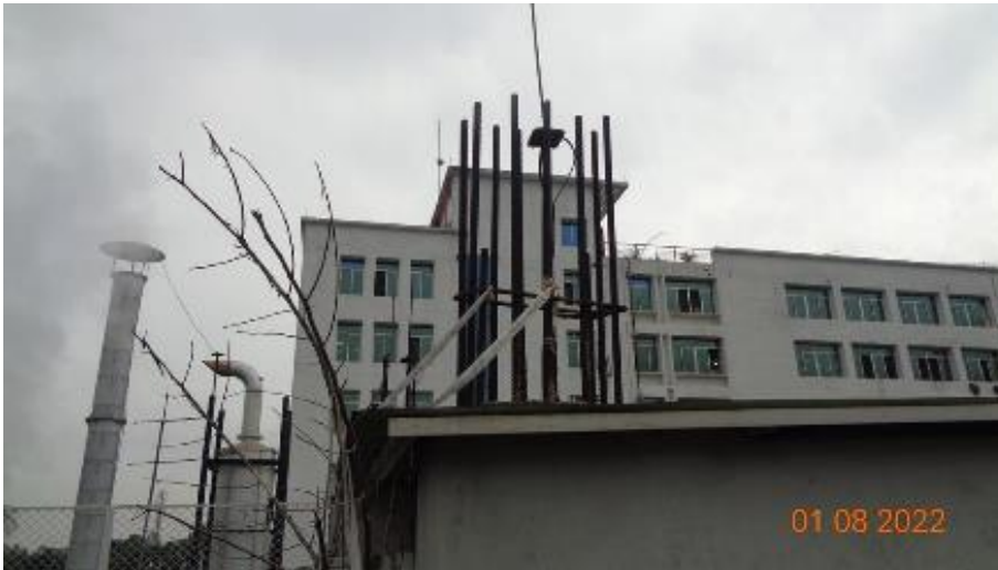
Corroded rebar on roof.
