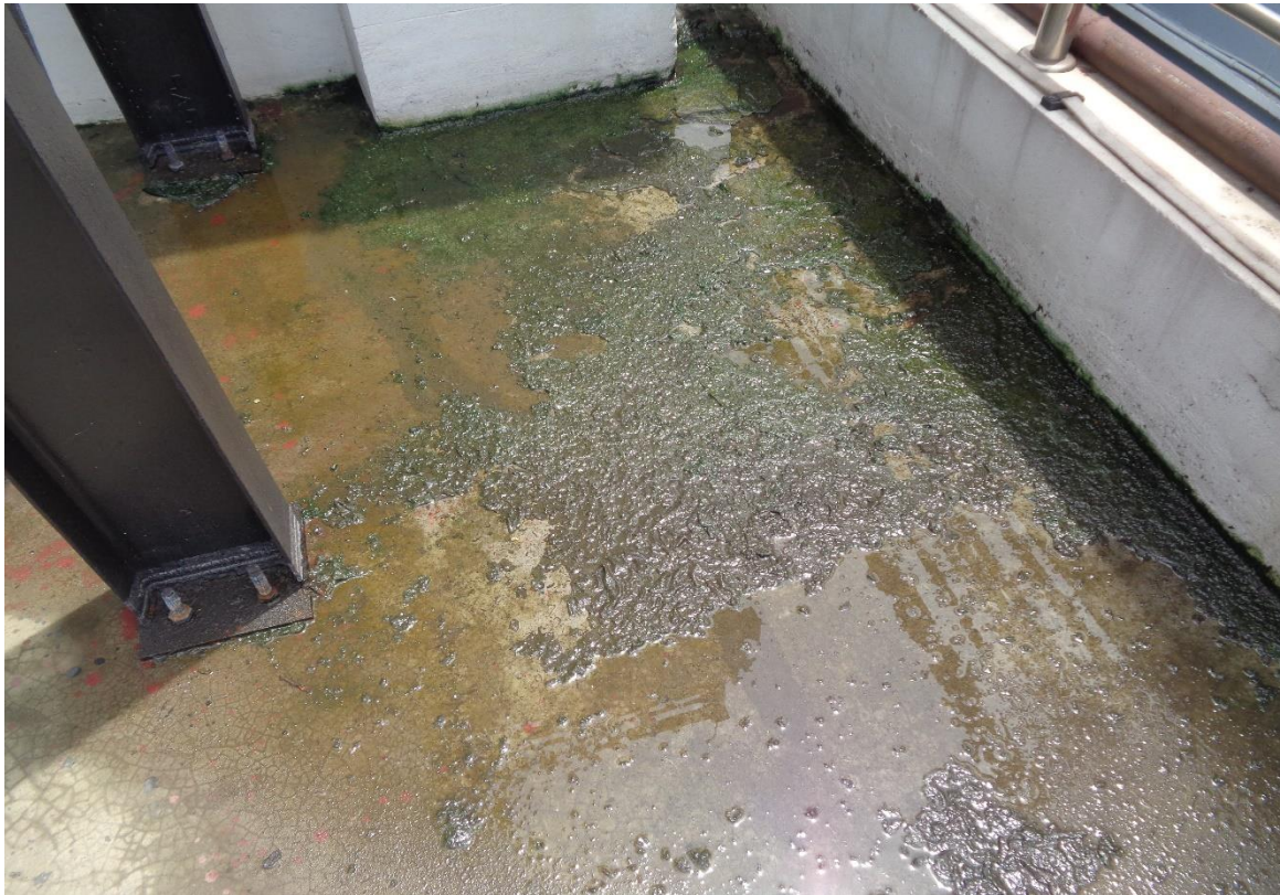
Water ponding on roof slab due to poor drainage system
