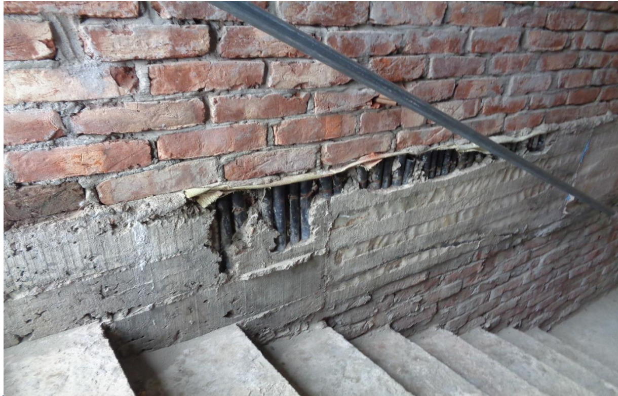
Ducting in beam at staircase area
