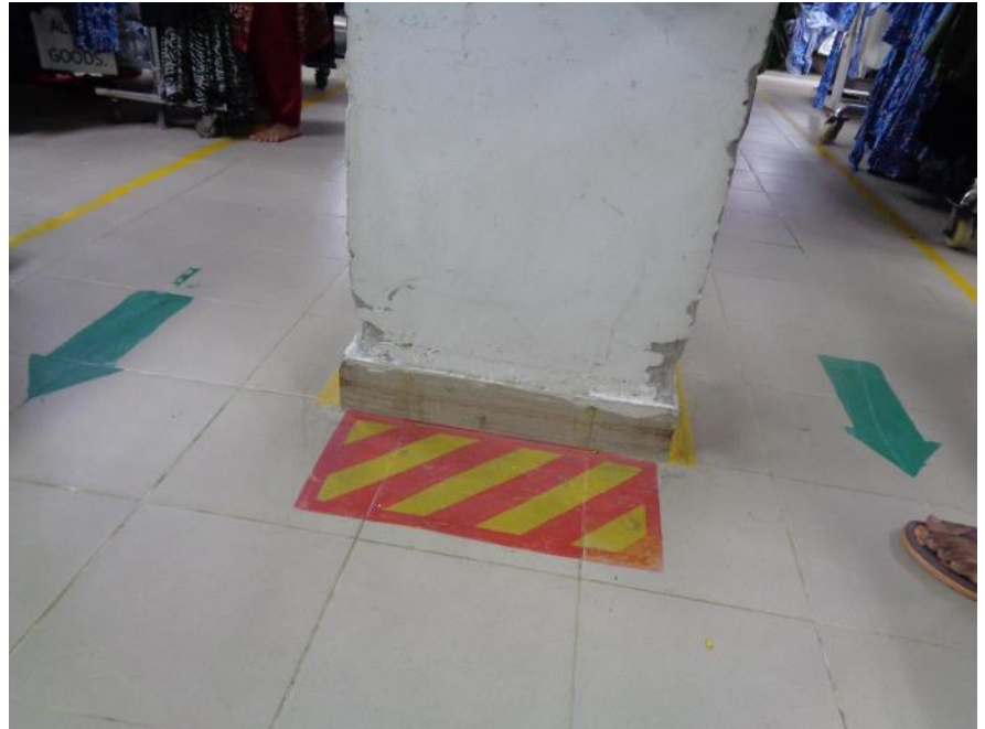
Column damage due to trolley impact in Building-2
