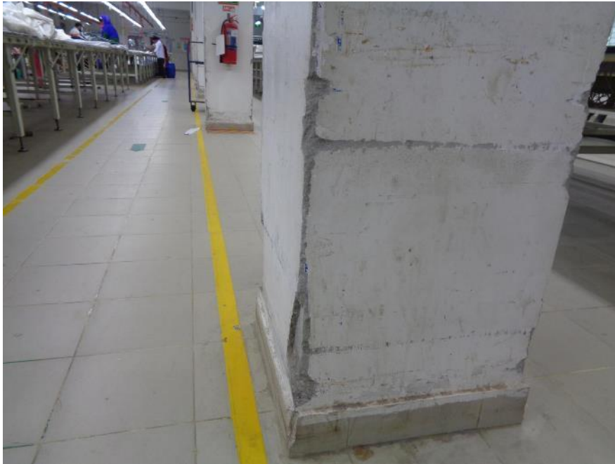
Column damage due to trolley impact in Building-2
